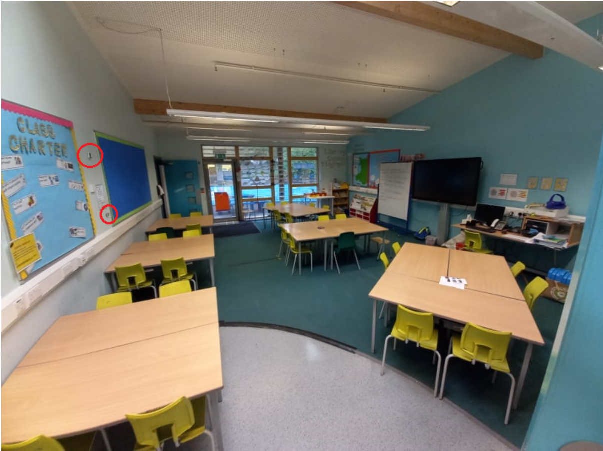
T/RH and CO 2 sensors in School A - classroom B
