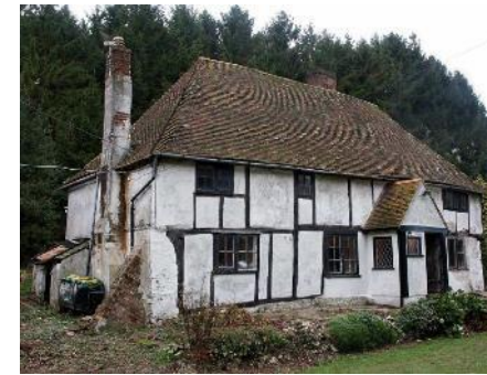
Close studding and Square framing Sources: DBRG 2008, CAS 2010
