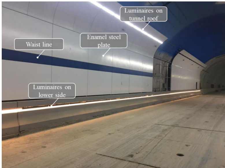
Fig.12 Installed luminaires and other facilities during construction
