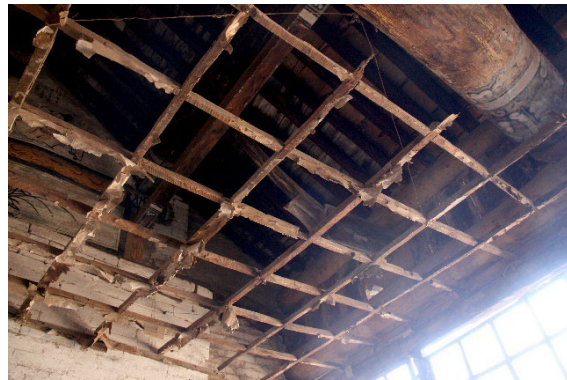
Figure 20 Frame of the added ceiling from the school period in the stage, as seen in April 2013 (Tam 2013f).
