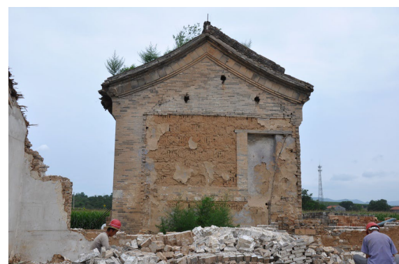
Figure 94 The west sidewall of the stage after the division wall was demolished, August 2012 (National Heritage Centre of Tsinghua University 2015)
