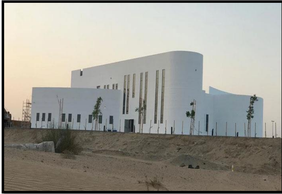
Figure 2-29 Apis Cor Largest 3D Printed Building.
