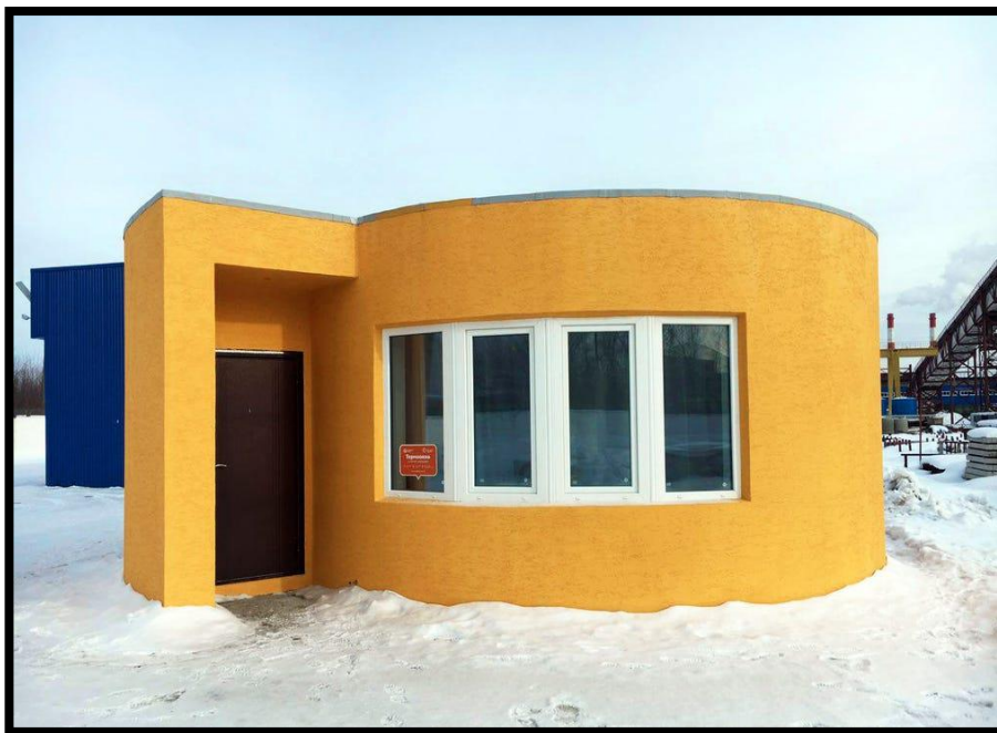
Figure 2-28 Apis Cor 3D Printed House (Garfield 2017).
