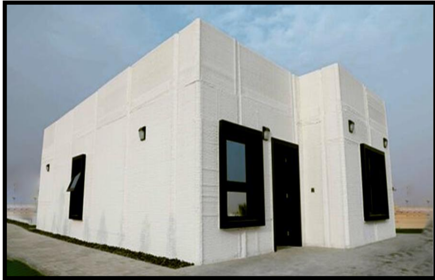
Figure 2-25 3D Printed House in Saudi Arabia (Ministry of Housing 2018).
