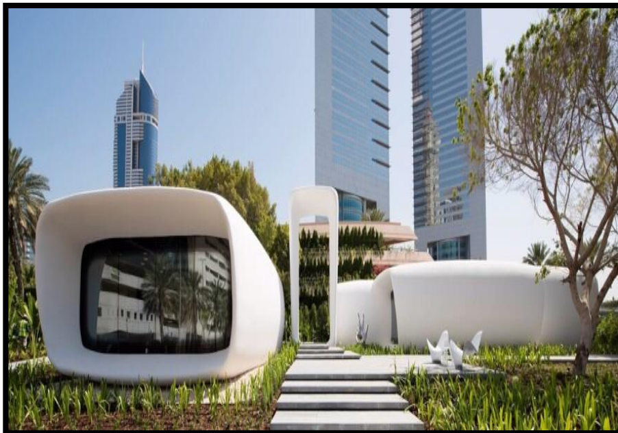
Figure 2-23 The 3D Printed Office Building in Dubai (Busta 2016).
