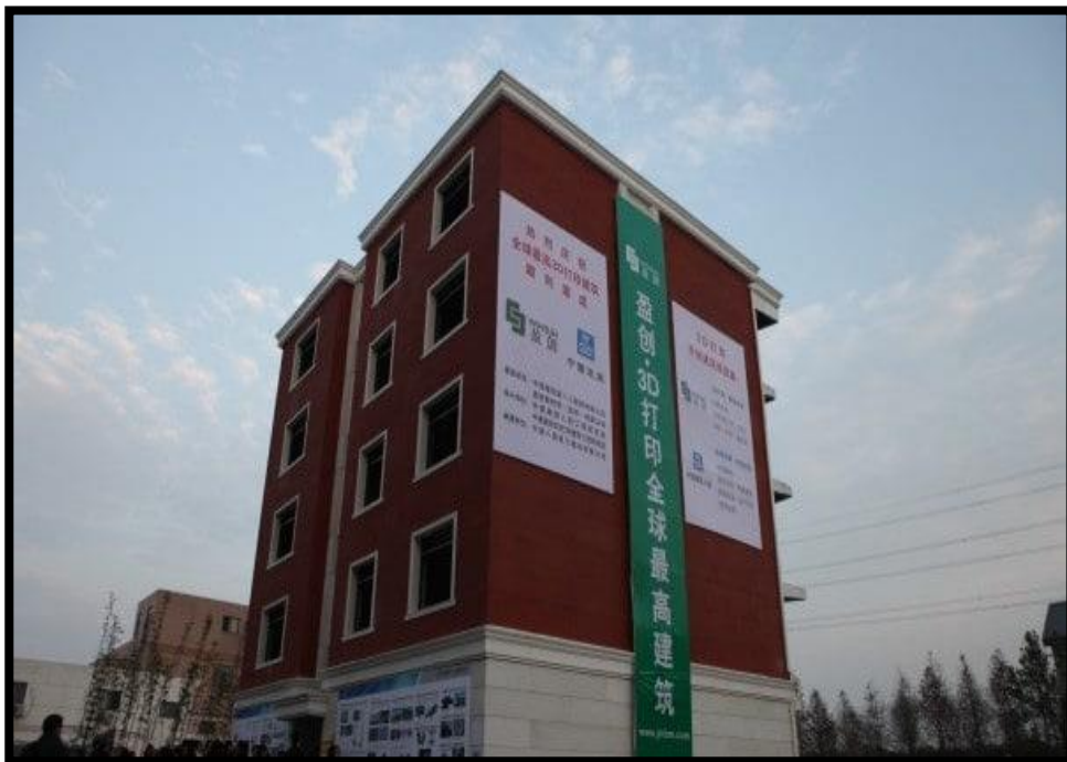
Figure 2-22 The Tallest 3D Printed Building in the World.
