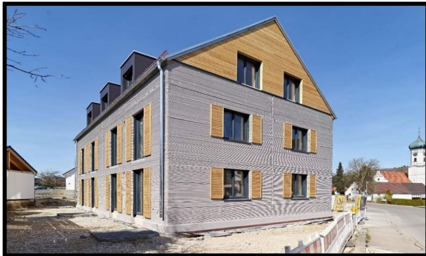
Figure 2-32 Europe's Largest 3D Printed Apartment Building (PERI 2021).
