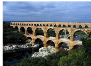
The Roman aqueduct Pont du Gard , France. The upper tier encloses an aqueduct which carried water to Nîmes in Roman times; its lower tier was expanded in the 1740s to carry a wide road across the river
