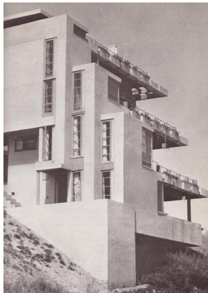
Figure 2.10: Wolfe House (Source: https://esotericsurvey.blogspot.com/2014/10/shnidler-bonhams.html , Accessed: 13 June 2019)
