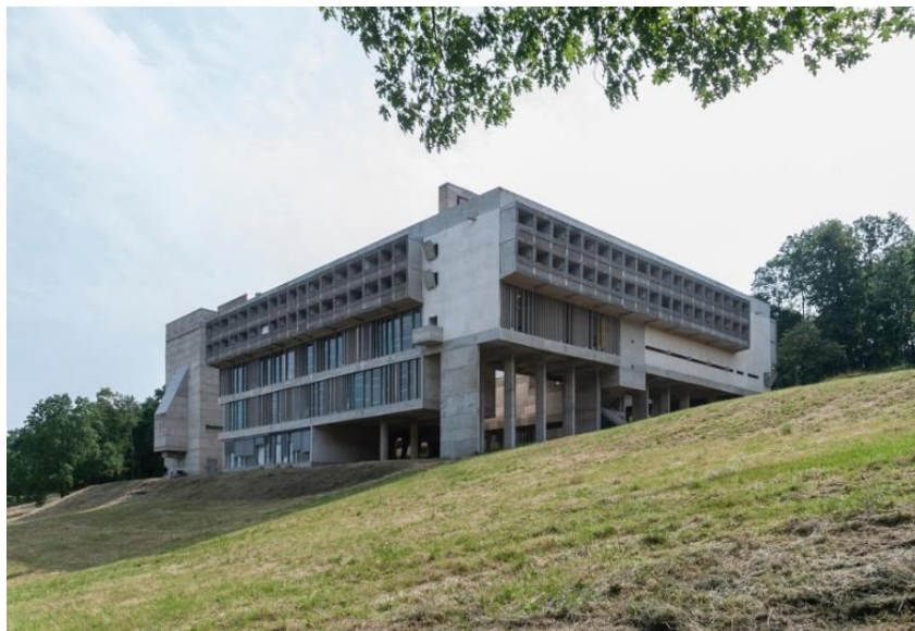
Figure 2.12: La Tourette, Le Corbusier (Source: https://www.archdaily.com/96824/ad-classics-convent-of-la-tourette-le-corbuier , Accessed: 13 June 2019)
