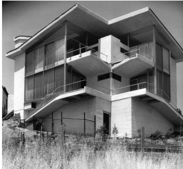
Figure 2.11: Van Patten House (Source: https://www.cosmicinspirocloud.com/post/124514699157/r-m-schindler-van-patten-house-moreno-drive , Accessed: 13 June 2019)
