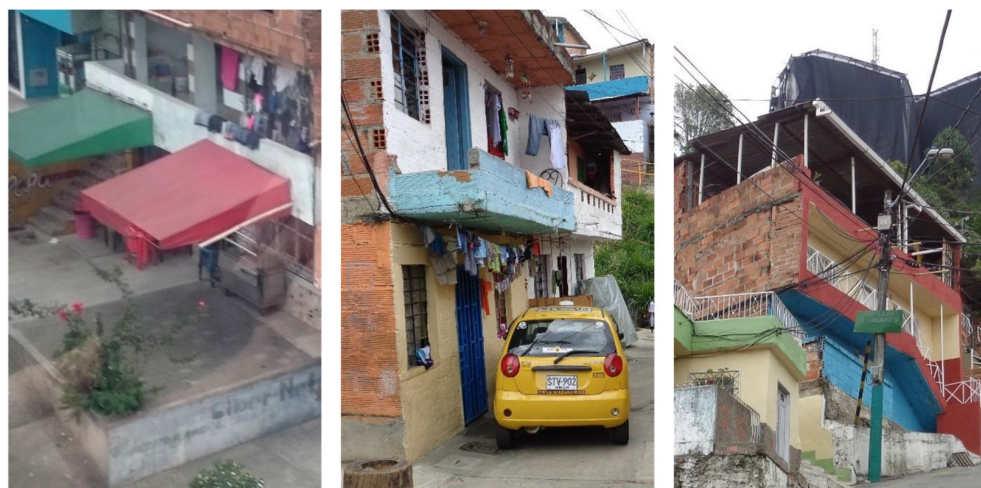
Figure 10. Extending the existing structures by adding a roof terrace (right), a balcony (middle), or a veranda (left). Photos: Hesam Kamalipour.
