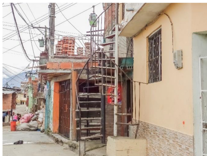
Figure 11. Dividing units by adding external staircases. Photo: Hesam Kamalipour.
