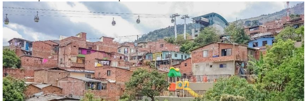
Insertion of a cable metro system that is integrated with the metro system of the city
