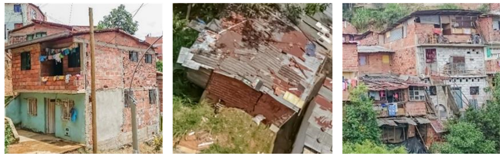
Figure 8. Construction materials: a building with temporary materials next to a building with a vertical mix of temporary and permanent materials ( right ); an informal structure with temporary materials along a creek ( middle ); a house with durable construction materials ( left ). Photos: Hesam Kamalipour.
