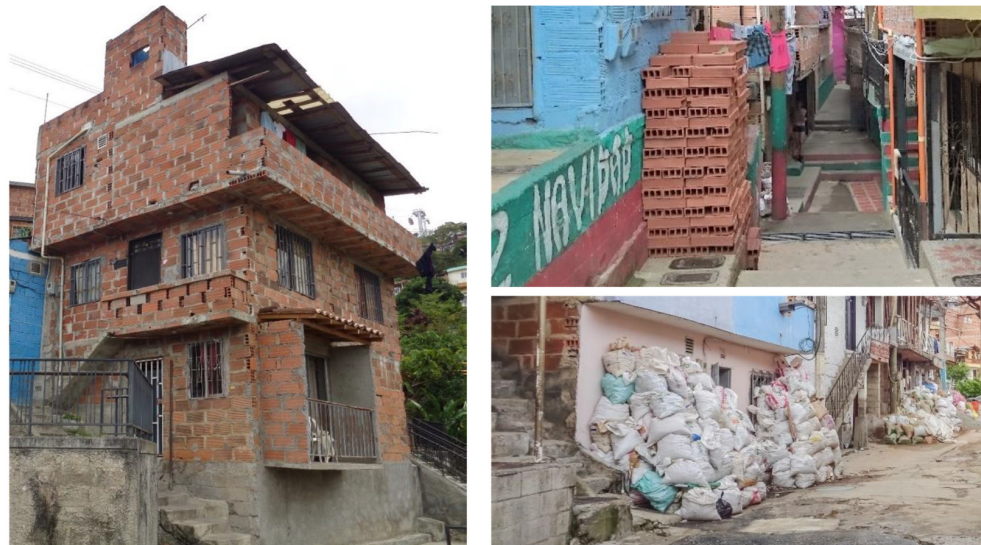
Figure 9. Adding multiple rooms: adding permanent rooms (left); storing materials against a blank wall (upper right); storing material in front of a house (lower right). Photos: Hesam Kamalipour.
