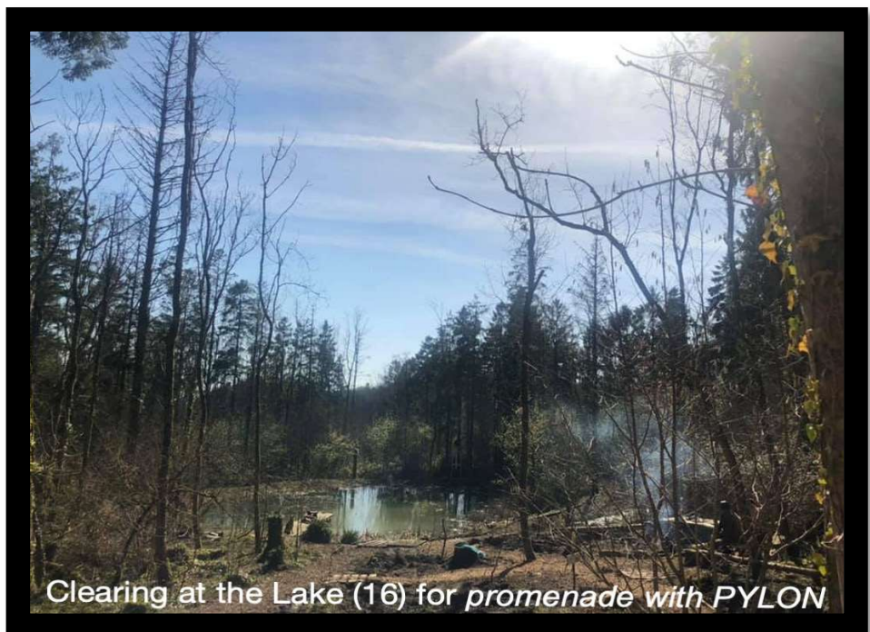
Figure 20: Clearing at the Lake for promenade with PYLON. Photo by author (2019).
