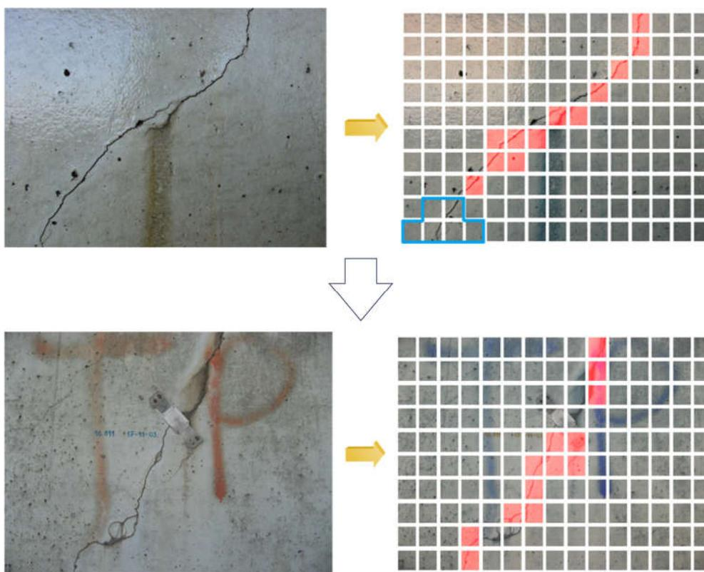
Fig. 5 Few-shot crack detection in real bridge inspection images
