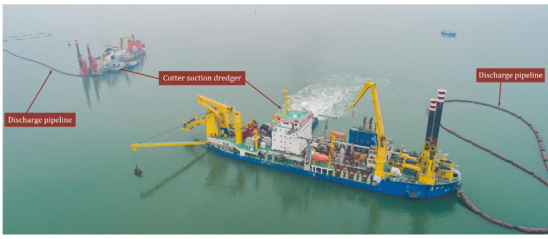
Fig. 1. The excavating process of cutter suction dredgers.
