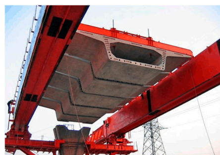
Figure 1. Rapid construction of segmental precast box girder.
