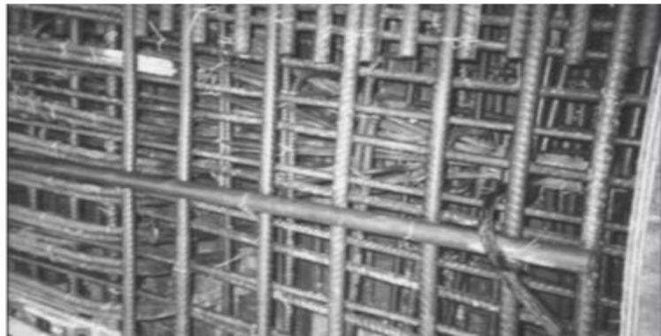
Figure 2.1: An example of congested reinforcement, an ideal application for SCC (Goodier and Repository, 2003)
