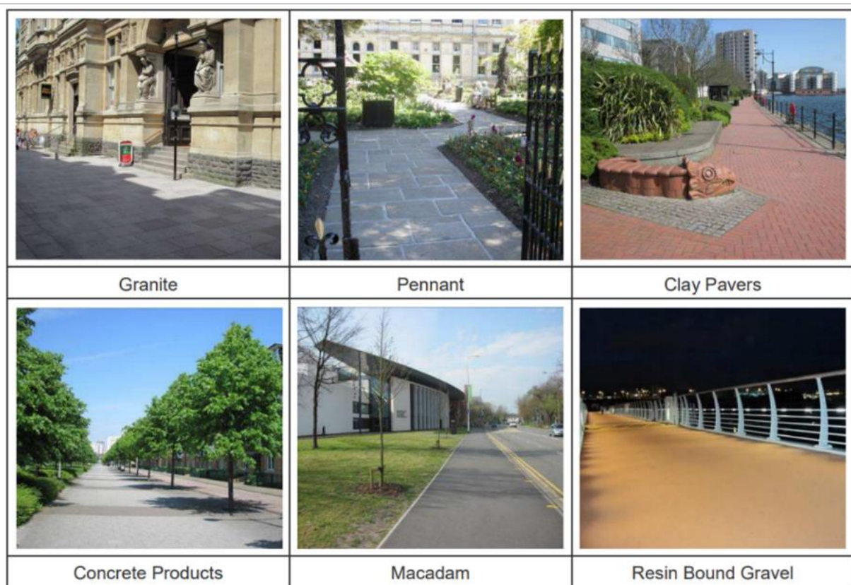
Figure 2: Example Images of Footpath Paving Materials (images from Cardiff Public Realm Manual).
