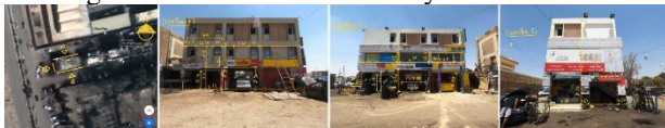
Figure 2. To the left is the location of the building, the western façade of the building, to the right the northern and southern façades of the building
