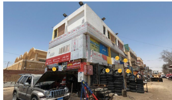
Figure 3. The workshop building with the six work places to be monitored.
