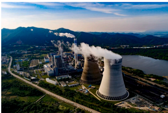
Fig. 18. Tongling power plant, anhui province, China [109].
