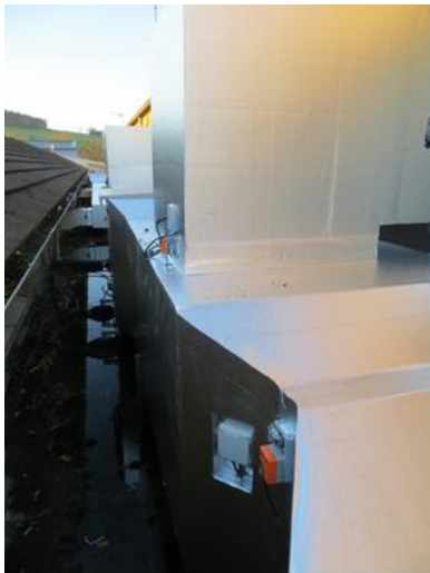
Figure 7-33 Lampeter cloakrooms; external duct installation and insulation (left) and supply grills integration (right), author.
