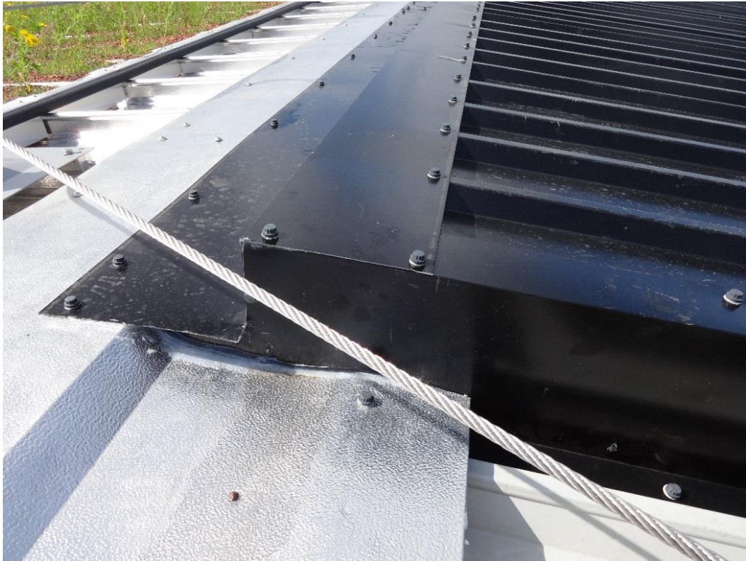
Figure 65. The detail linking the TSC panel to the ridge of the B&Q roof, author.
