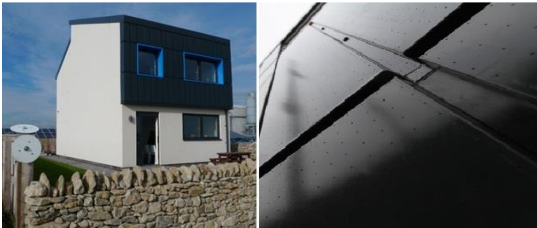
Figure 57. South wall façade integrated TSC (left) and detail of the metal cladding and perforation (right) at Solcer house, Wales, UK; author.
