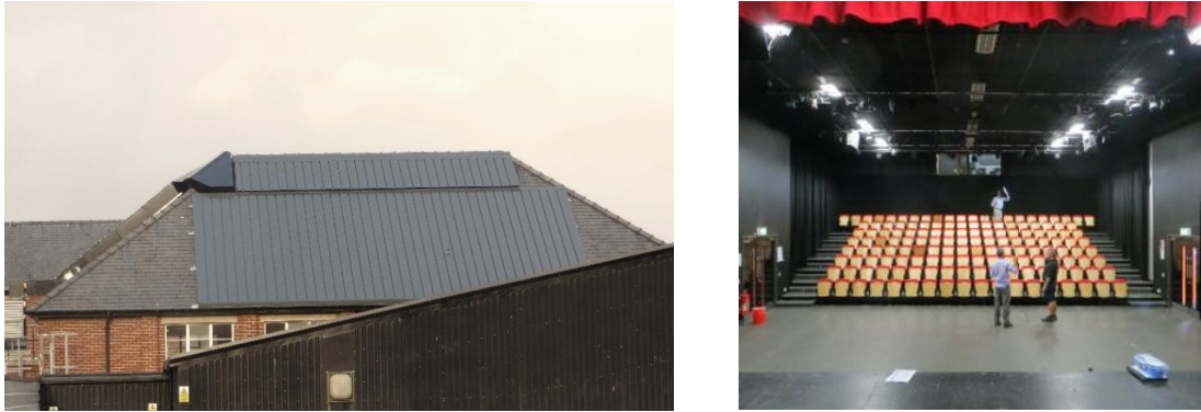
Figure 49. Inclined roof TSC (left) and delivery room - theatre (right) at Glan Clwyd School, St Asaph, Wales, UK; author.
