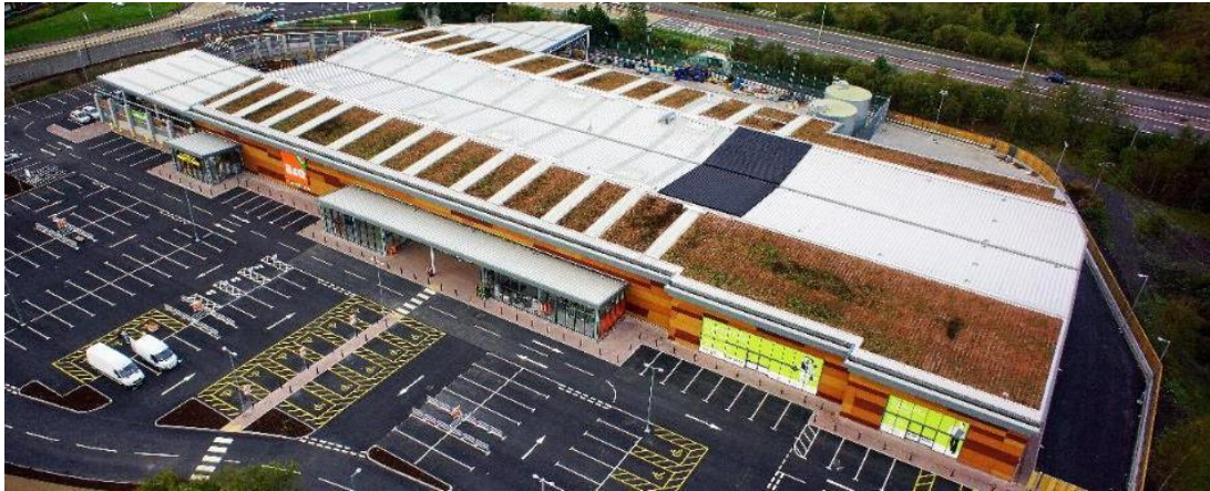
Figure 42. Roof-top TSC at B&Q Store, Merthyr Tydfil, Wales, UK; WSA team
