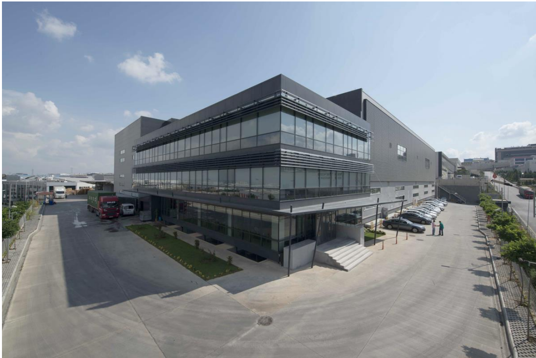
Figure 30. The TSC installation on the south facade of PIMSA Automotive production plant in Turkey (22).
