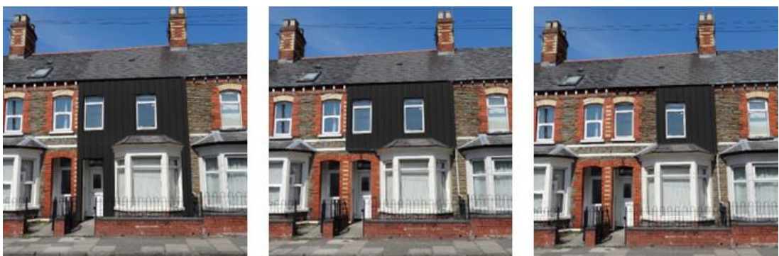
Figure 6-12 Images showing the TSC in three variations of elevation area. From left to right: whole façade, half façade, ¼ of façade, SBED project including the author.
