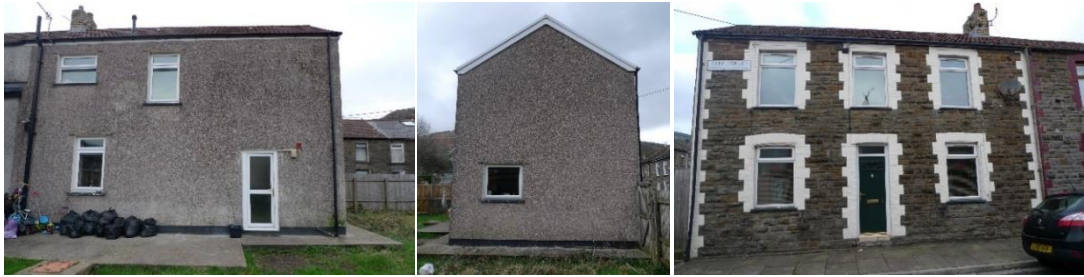
Figure 7-5 Rhondda end-terraced house; From left to right, west, south and east elevation, author.
