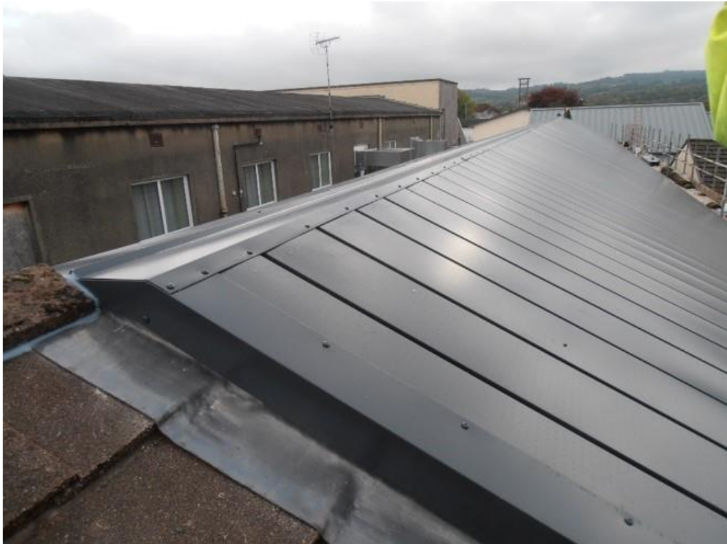
Figure 63. The finished 'Lampeter TSC' installation from up close, author.
