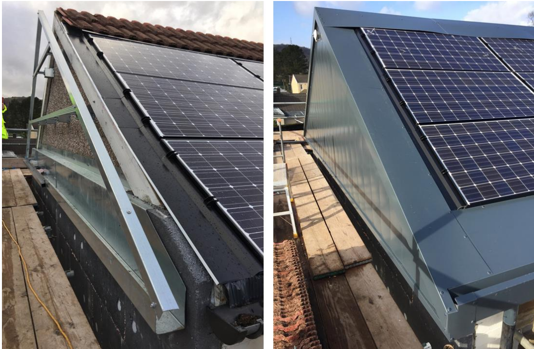
Figure 7-29 Rhondda end terraced; TSC supporting structure (left) and end-product (right), author.
