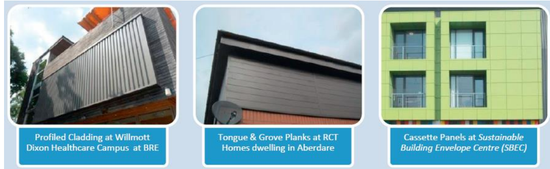
Figure 3-6. Examples of the three types of metal cladding available for TSCs (69).
