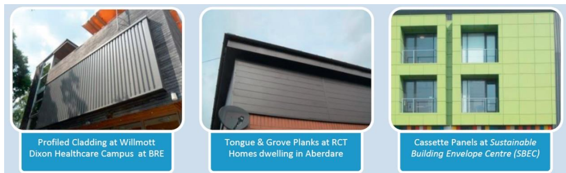
Figure 6-9. Examples of the three different types of metal cladding available for TSC (69).
