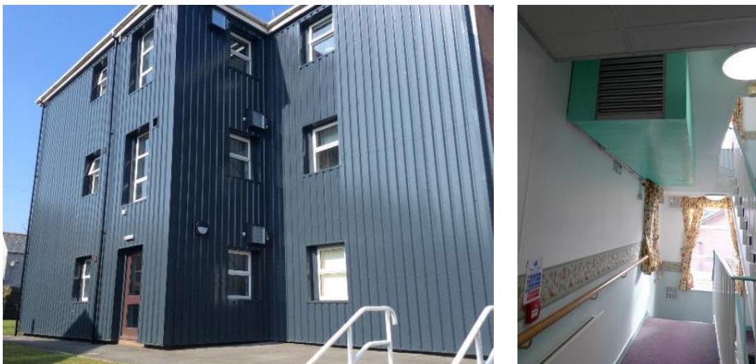
Figure 53. Vertical wall with two TSC south facing facades and one “dummy” east facing façade (left) and one of the three delivery corridors on the 1st floor (right) at Saxon Court residence, Ebbw Vale, Wales, UK; author.
