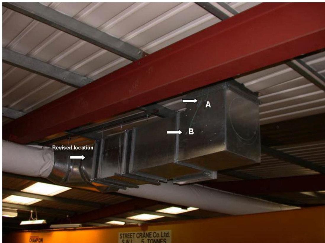
Figure 24. Location of thermocouples within building (17).
