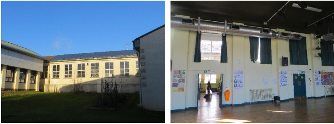
Figure 46. Inclined roof TSC (left) and main hall distribution duct (right) at Lampeter School, Ceredigion, Wales, UK; author.
