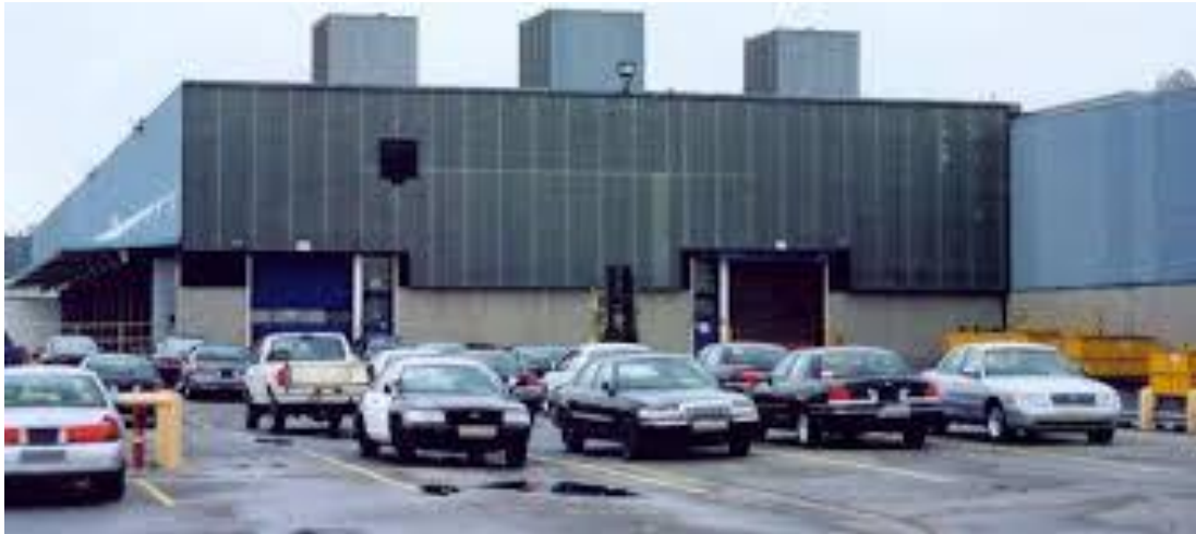
Figure 2. Part of the TSC installation at the Ford Assembly Plant in Ontario, Canada (3).
