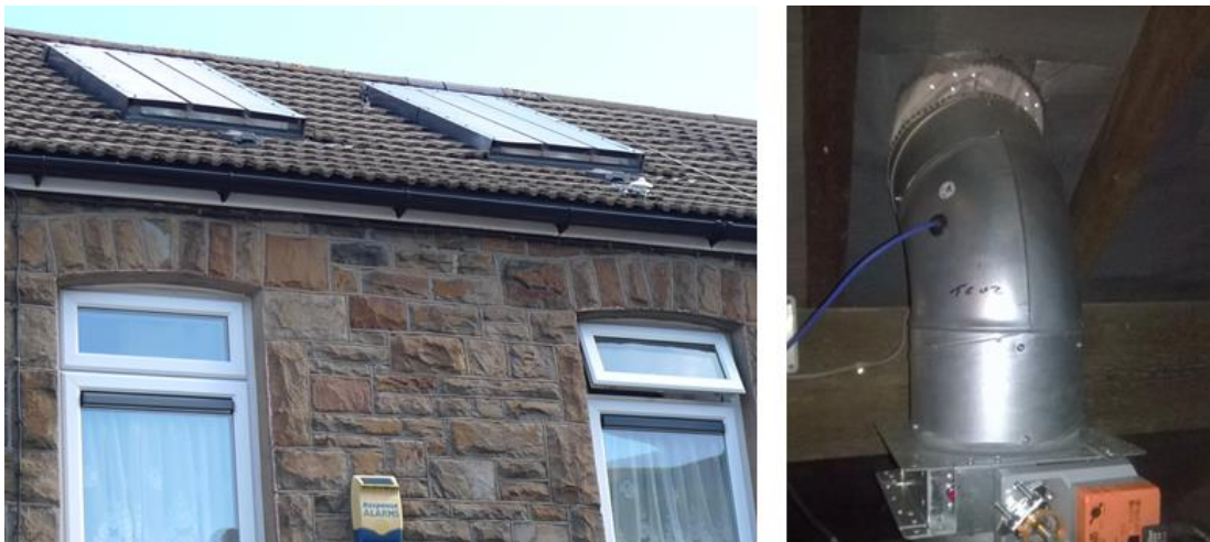
Figure 7-32 Rhondda terraced; roof integration (left) and duct inlet (right) during installation, author.
