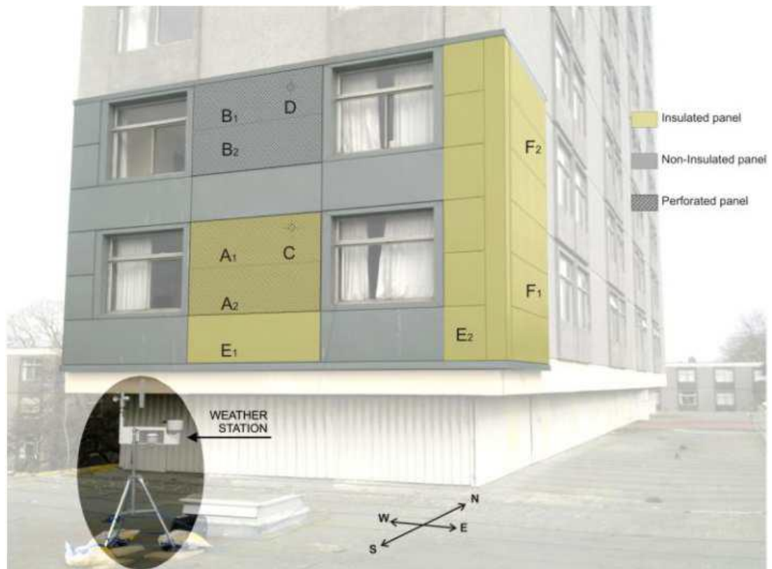
Figure 39. Insulated, non-insulated and perforated panels on south and east façade of the building in Wheatley campus (24).
