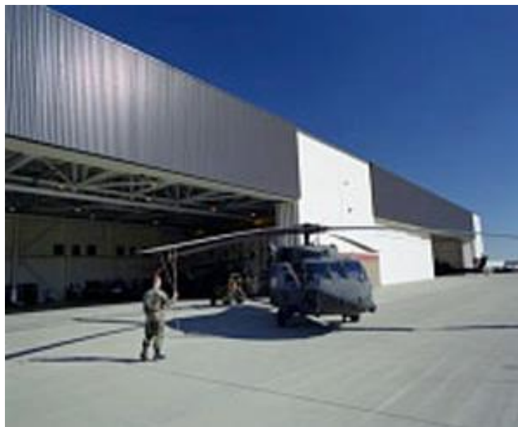
Figure 15. TSC installation on the US Army Hangar, Colorado, U.S. (6).
