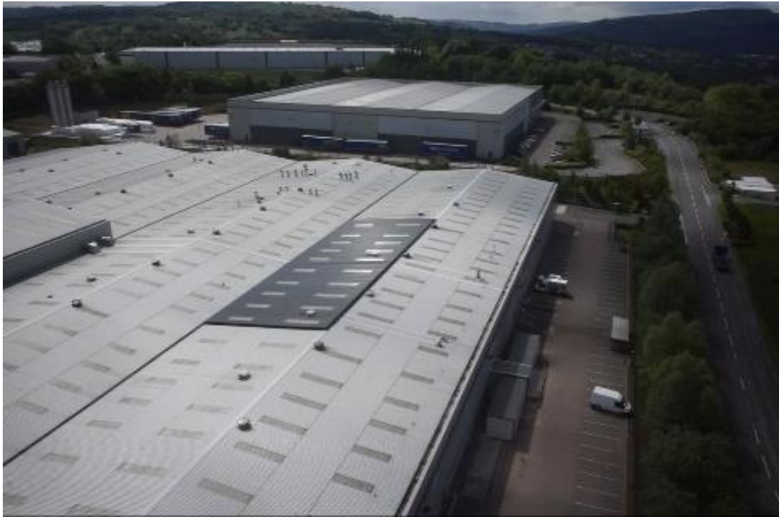
Figure 44. Roof-top TSC at SEDA UK Ltd. Blackwood, Wales, UK; author. Note: the TSC is the black panel area.
