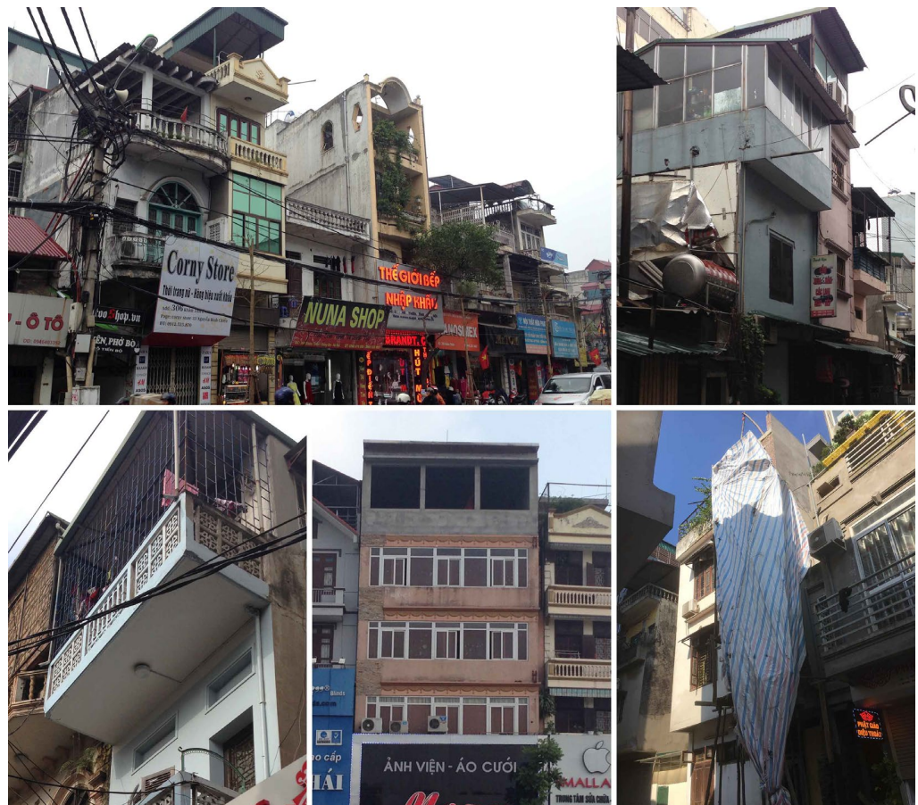
Figure 9. Diverse architectural styles of buildings ( upper left ); a temporary structure added over the top of a building to increase living space ( upper right ); a contemporary structure added over the balcony ( lower left ); the addition of a new storey ( lower middle ); a new house built over the site of an old building ( lower right ).
