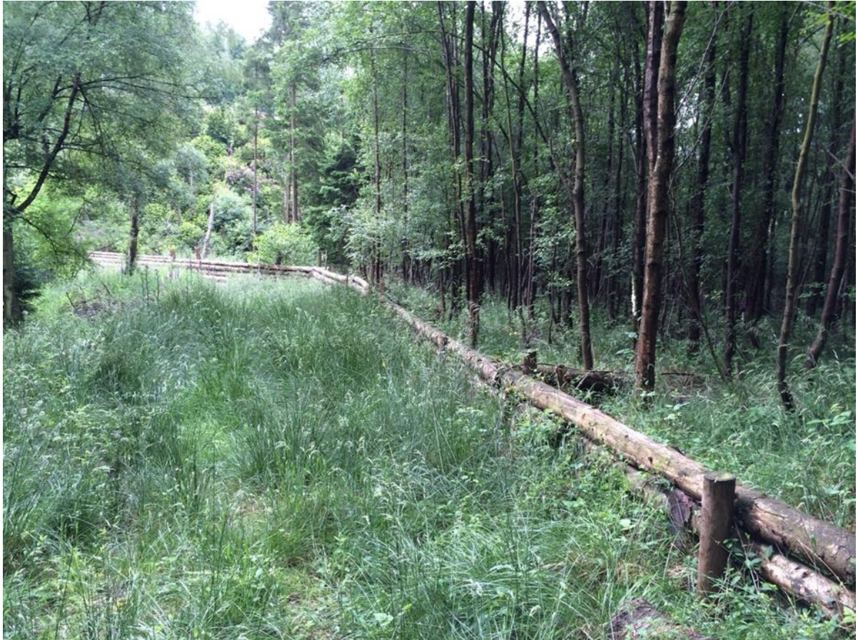
Figure 6.34: Photograph displaying a WDD that spans the floodplain at Pickering (Peak Chief Executive, 2016).
