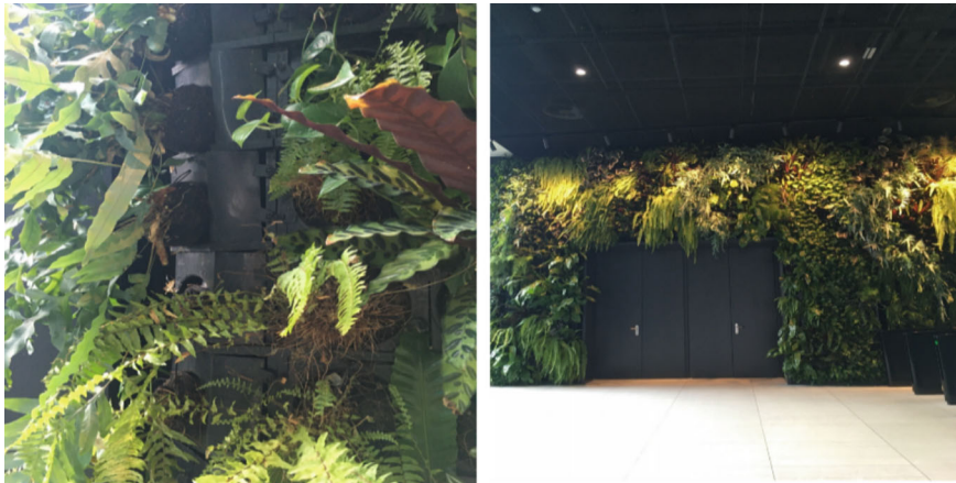
Fig. 8.4 Indoor modular system of the vertical garden WallGreen in an office building (Porto Office Park, Porto-Portugal). Credits: Cristina Calheiros
