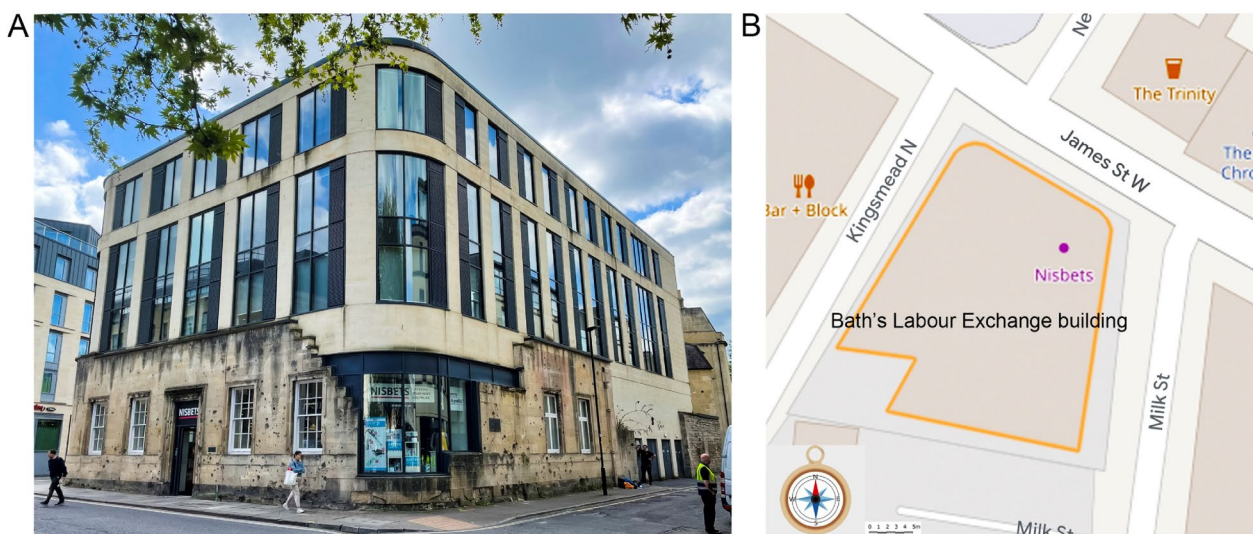
Fig. 2 A Labour Exchange building in Bath in 2022. B Geographical location of the building in Open Street Map [15]
