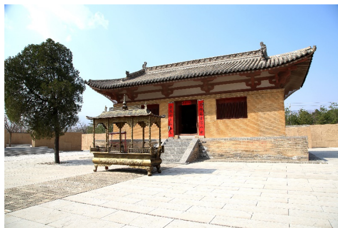
Figure 4. The main hall of Guangrenwang Temple after restoration, March 2018 (source: author).
