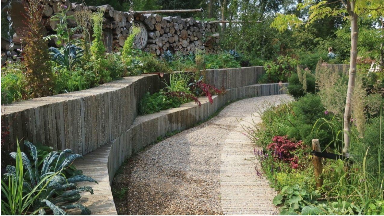
Figure 2.6: Concrete reuse for retaining walls. Diy garden projects, 2024 ( https://www.gardendesignstories.com/blog?tag=diy+garden+projects )
