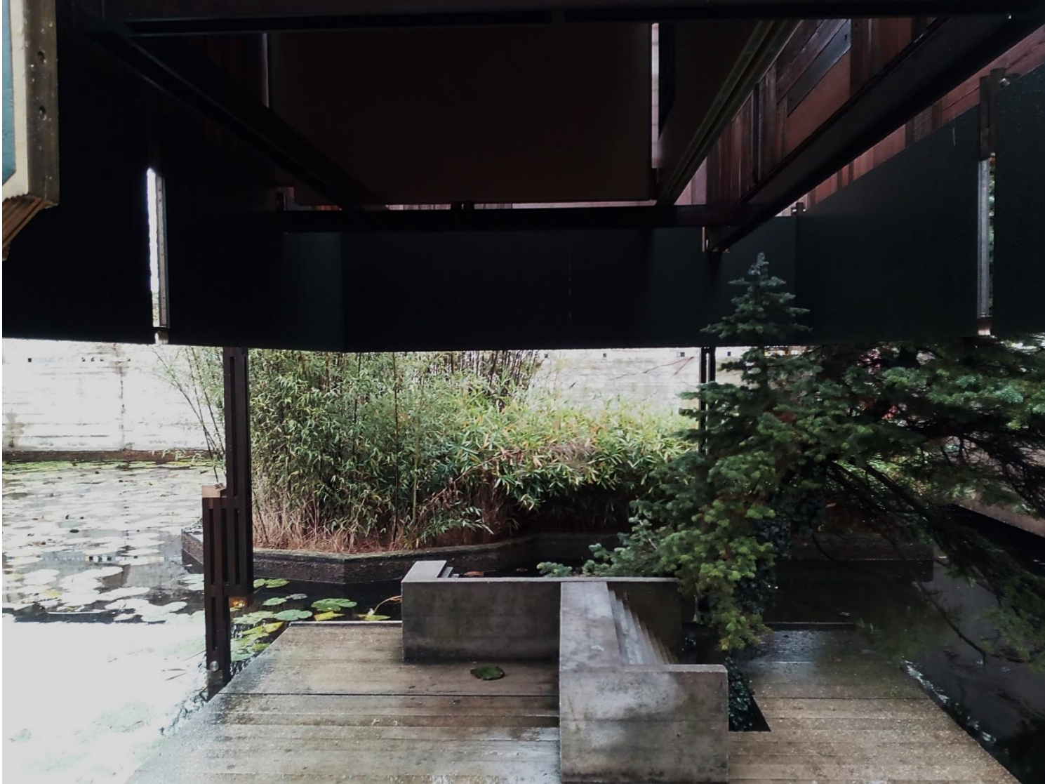
Figure 34 Inside the Water Pavilion, looking at the bench, the structure, and the panels above our heads
