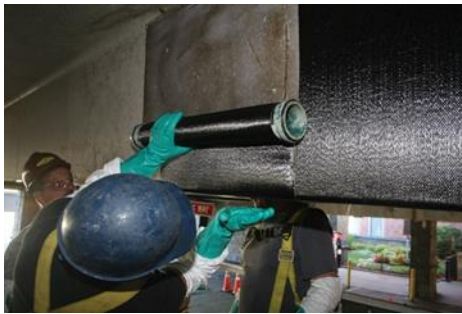
c) CFRP sheets installed around beams for shear stress
