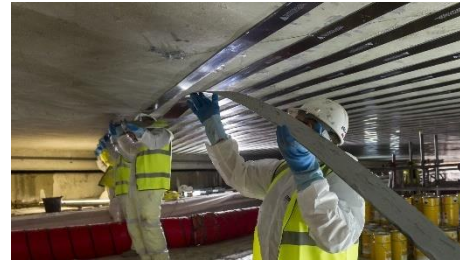
b) CFRP plates installed under a beam to gain flexural strength
