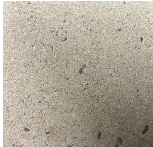
c) SP4 Level of surface preparation achieved
