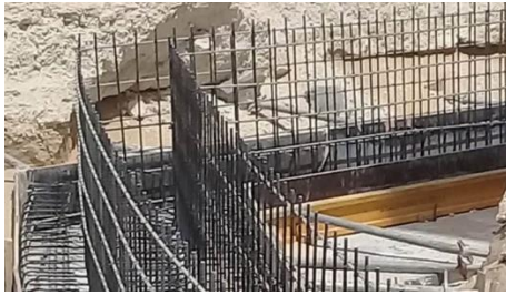
a) CFRP rods used in the construction of retaining wall
