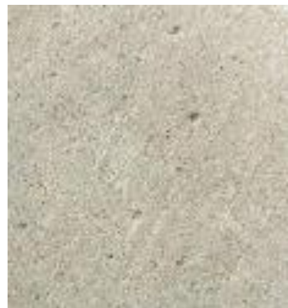
c) The surface preparation achieved from hand grinding the concrete
