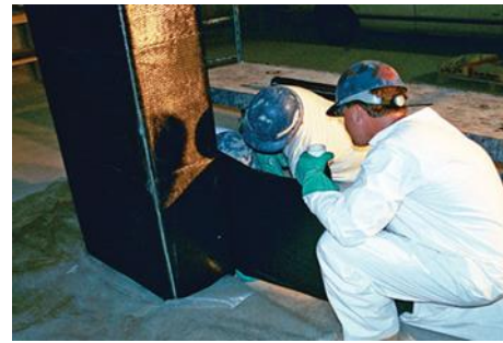
d) CFRP sheets installed around columns to increase compression capacity
