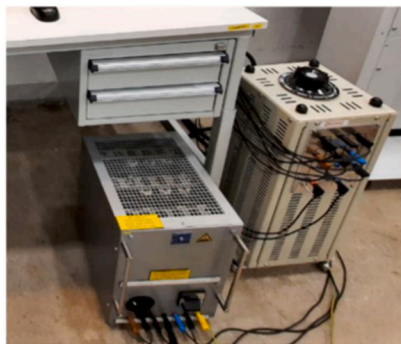
Electrical Load and Microgrid Connections
