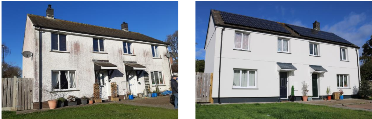
Figure 1 – Delivering a whole house energy system retrofit – before and after
