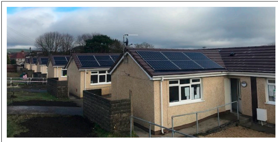
Figure 6. Six bungalows post-retrofit (CLCBE team).
