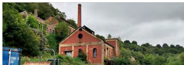
Figure 2: Crumlin Navigation Colliery (Whitman, 2021)
