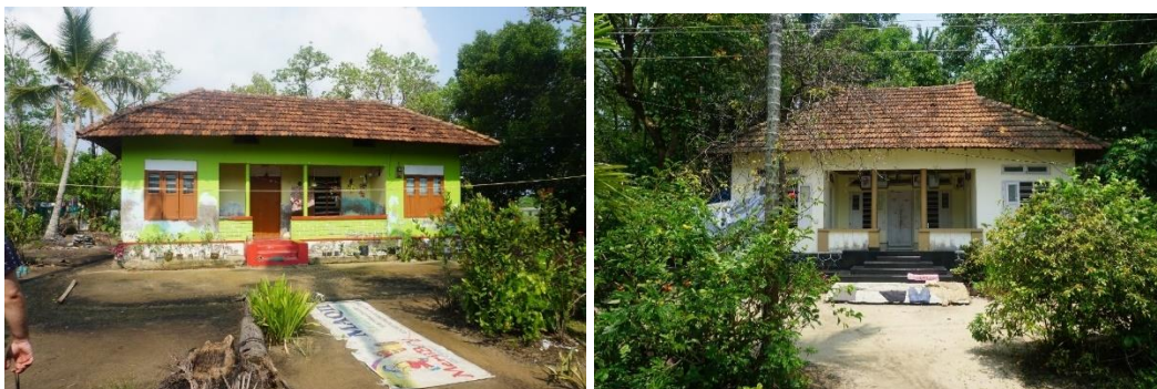
Figure 7. 13: Photographs of typical houses in the East Manjanakkad (above) and Cheriya Kadamakudy Island (below).
