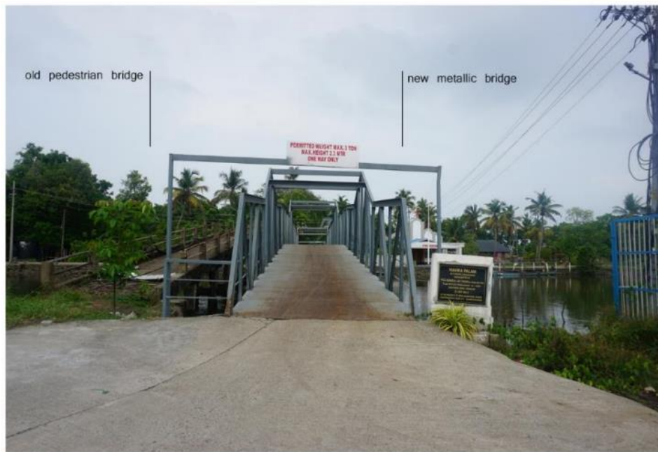
Figure 7. 23: Old pedestrian bridge and Navy's metal bridge in CKI.
