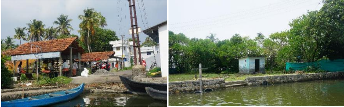
Figure 7.18: Manjanakkad Boat jetty providing access to EMI (left) and entrance area of EMI (right).
