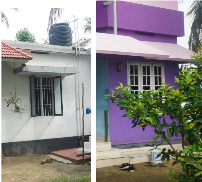
Figure 10.30: Windows protected by the eaves in EMI (left) and CKI (right).
