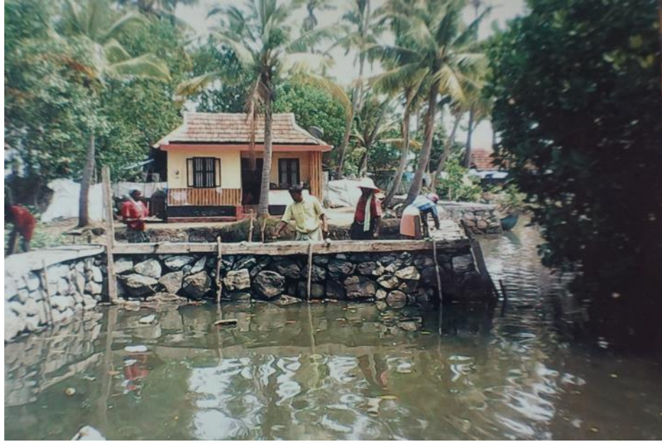
Figure 7.30: Photo showing the construction of the stone wall built by the government in the 1990s (source: archive of Dear Shobana living at EMI).
