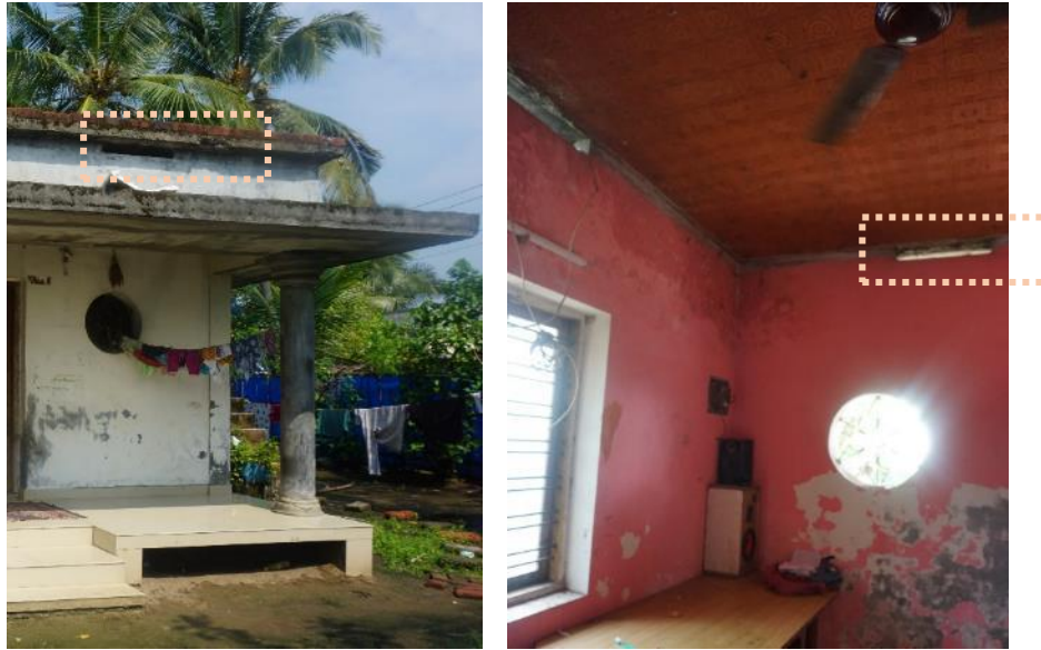
Figure 10.32: Example of ventilation window located under the roof in EMI.
