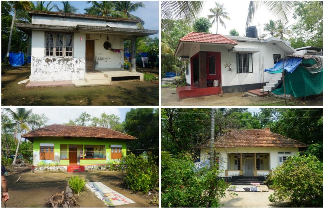
Figure 10.29: Flat roof with provision of eaves in EMI (upper right and left corners), hipped roof in EMI (bottom left corner), and hipped roof with ears in CKI (bottom right corner).
