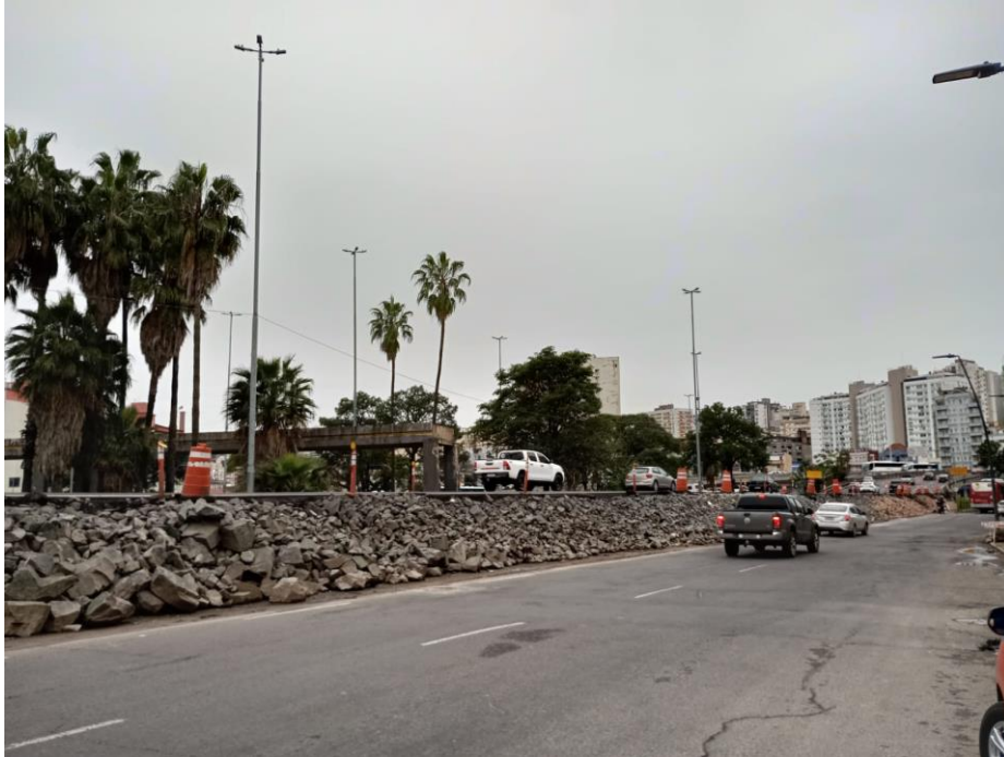
Fig. 4. Emergency Corridor structure in August 2024 (source: authors' archive).
