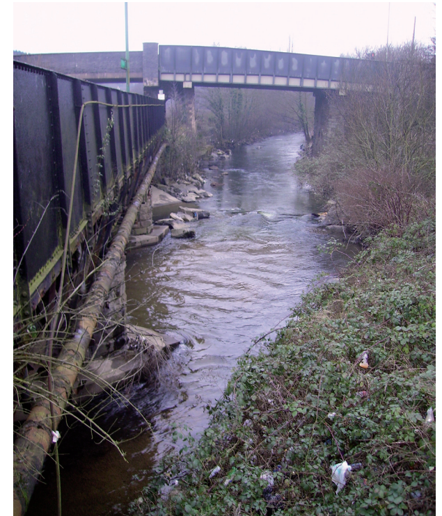
Fig. 35: View of the river to the edge of the Ton Pentre train station site (railway bridge to the left)
