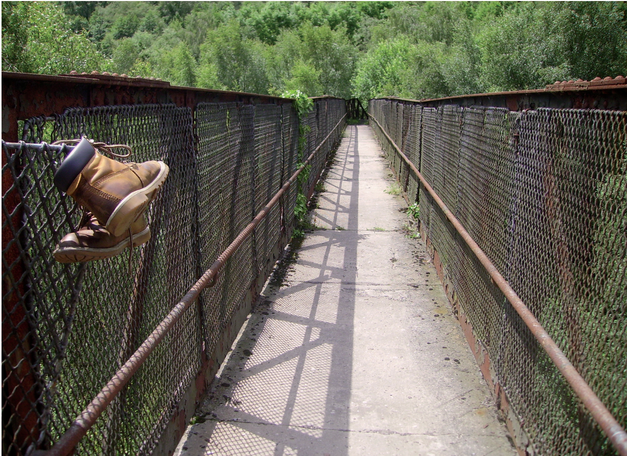
Fig. 11: 'Did he Jump' Pedestrian Bridge, Hopkinstown
