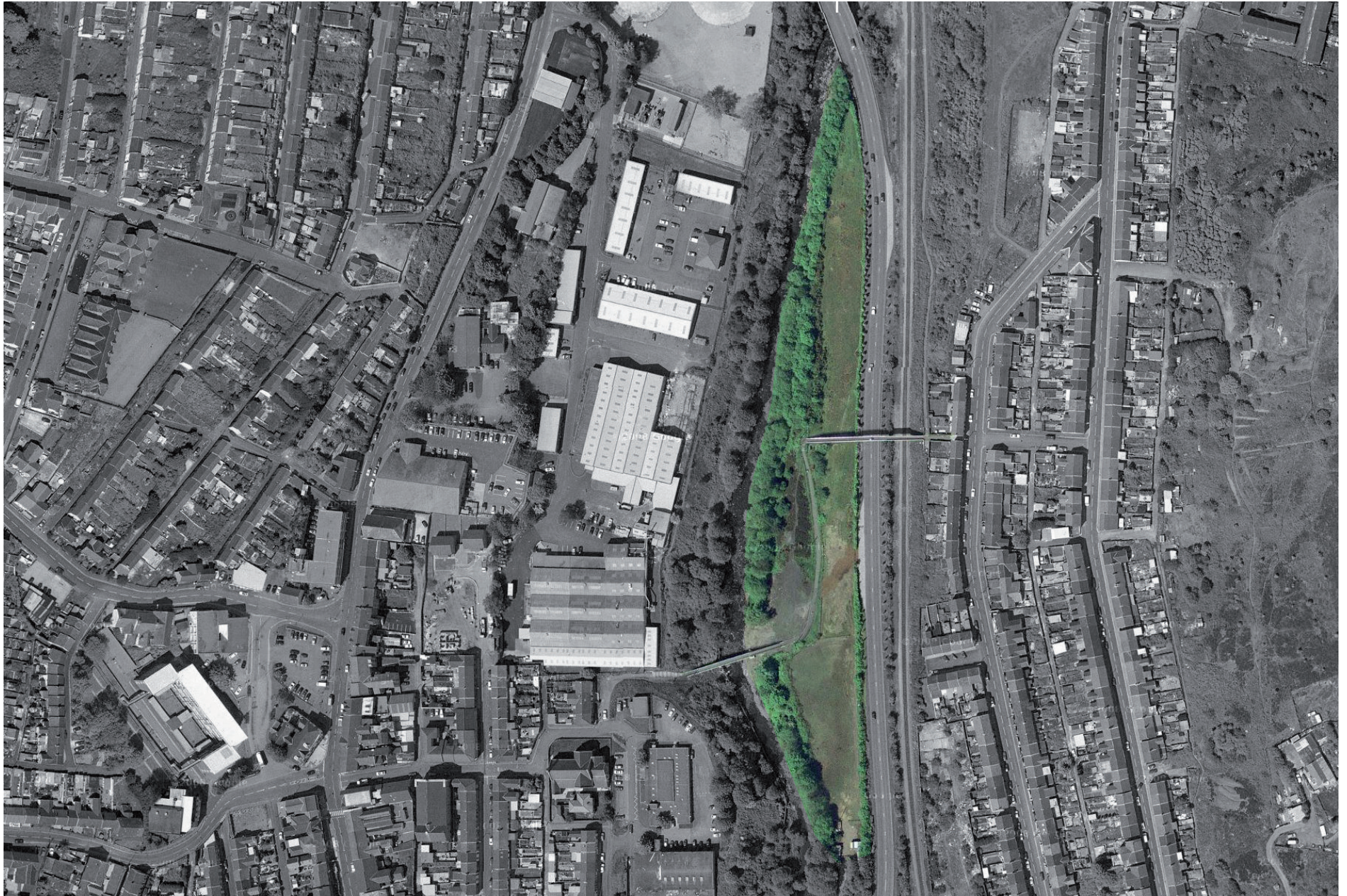
Fig. 8: Aerial view of #RS007 site
