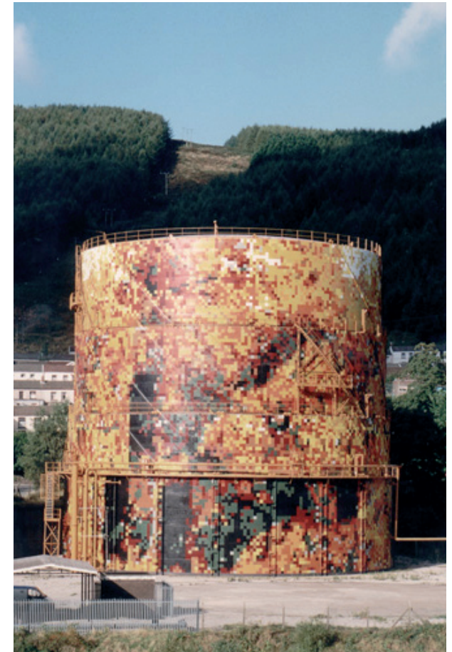
Gasometer & Valley context
