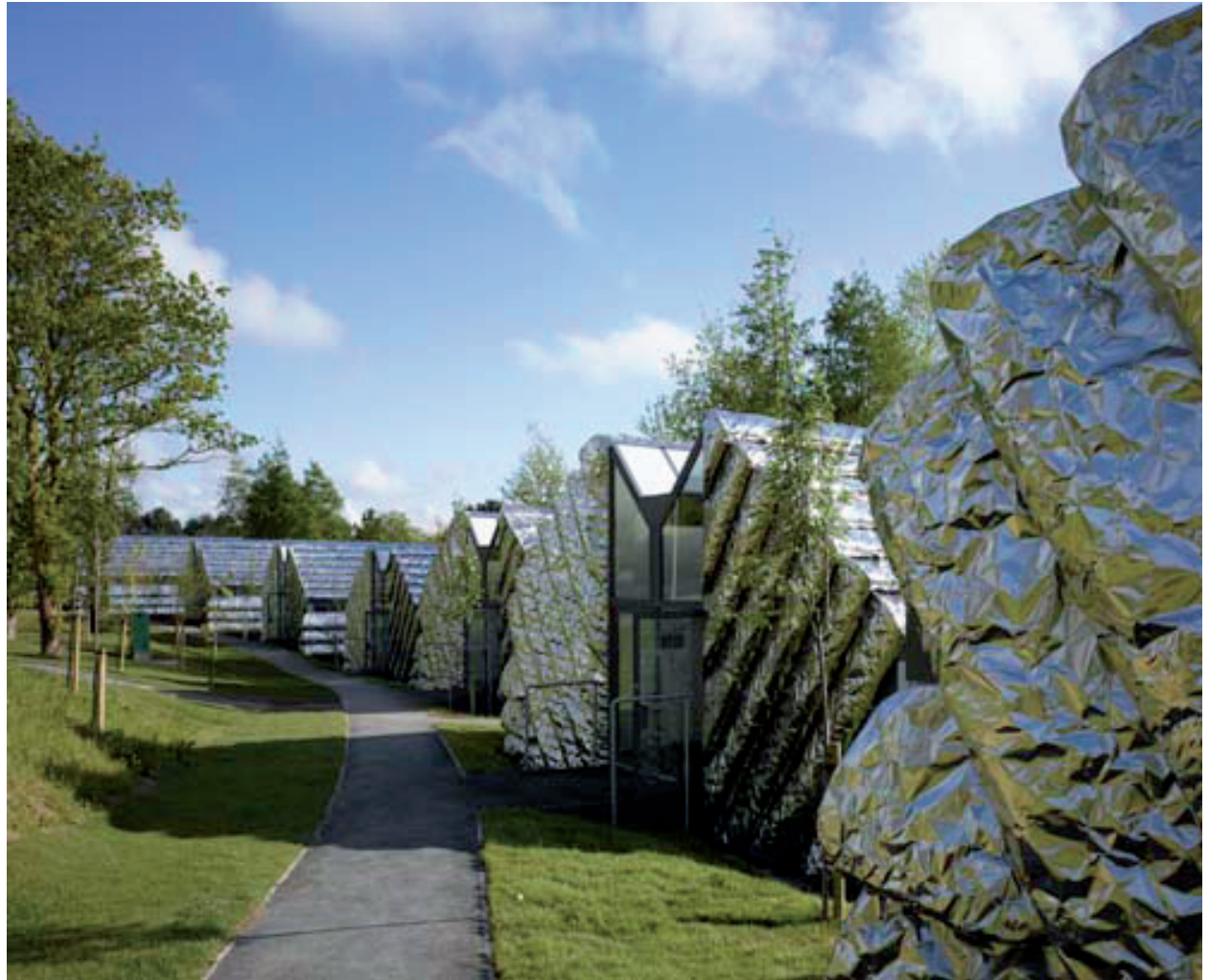
Fig. 27: Temporary allows testing of innovative cladding solution
