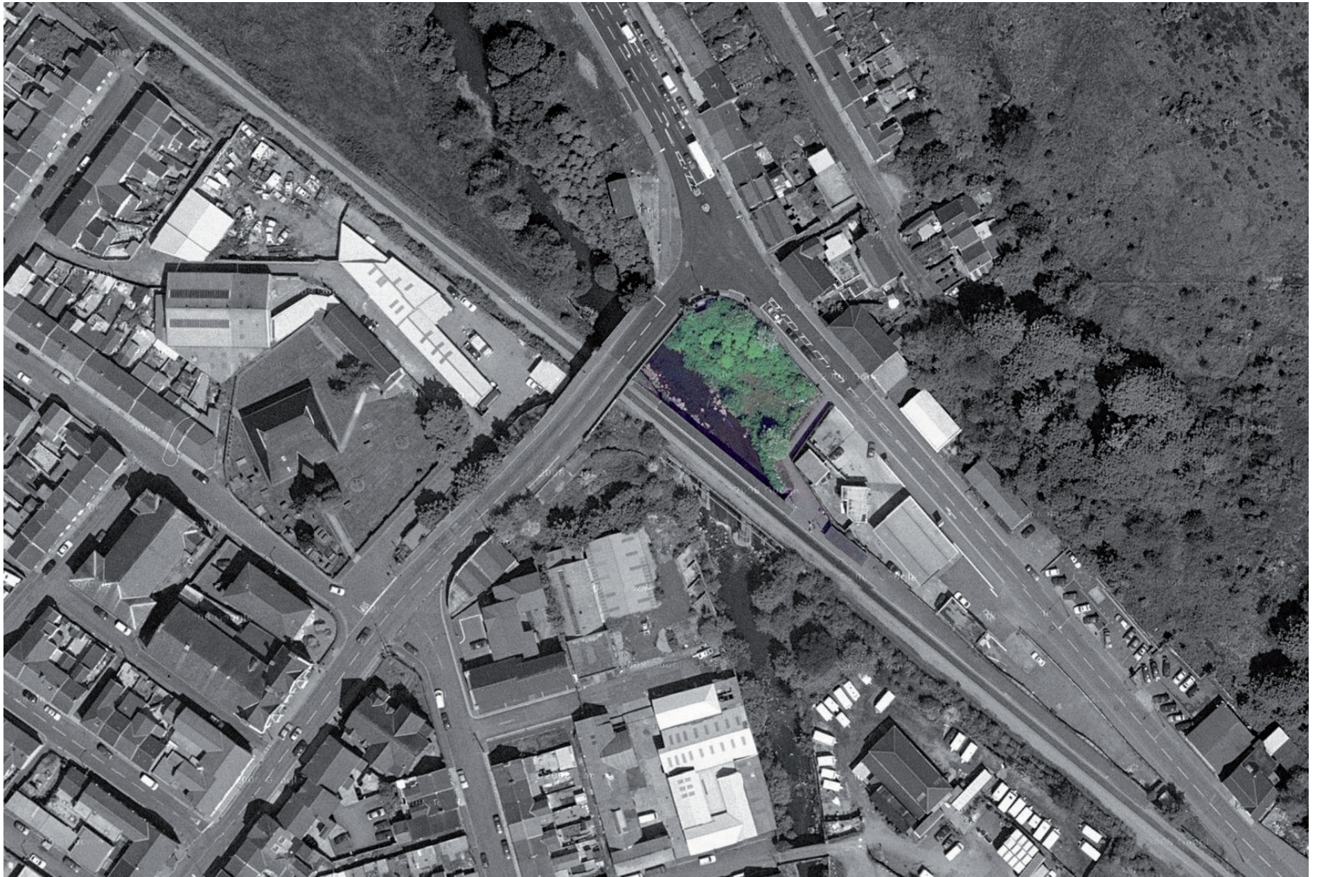
Fig. 10: Aerial view of #RS009 site
