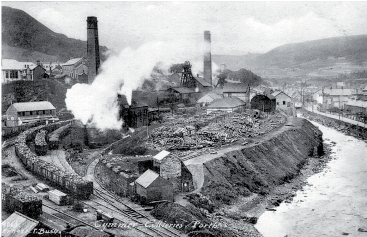
Fig. 22: 'Near-Exhaustion', Britannia and Lewis Merthyr Colliery II, Industrial Porth. The historical image illustrates the former 'Cymmer Colliery' position buried into the floor of the valley, slotted between the resource of the river and the once numerous coal transit train line networks.
