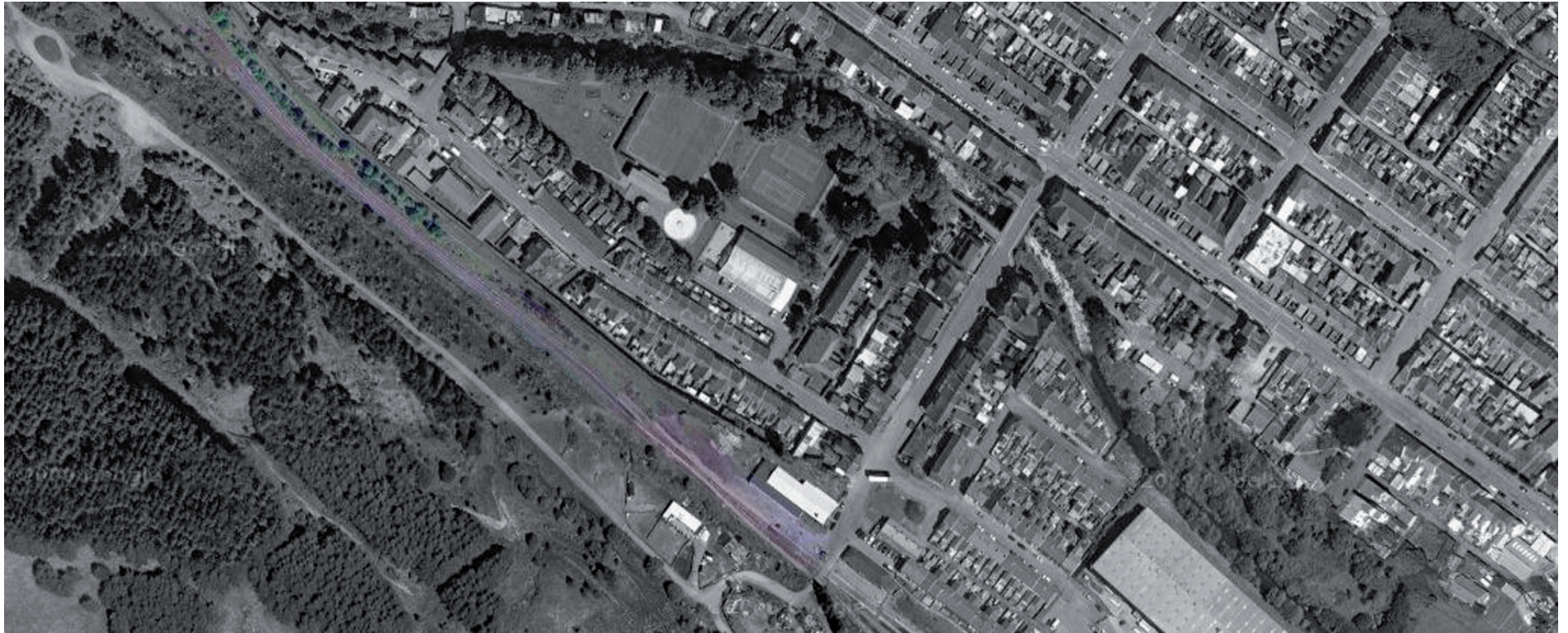
Fig. 12: Aerial view of #RS011 site
