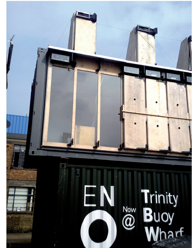
Fig. 25: Two-storey office from adapted shipping container, Trinity Buoy Wharf
