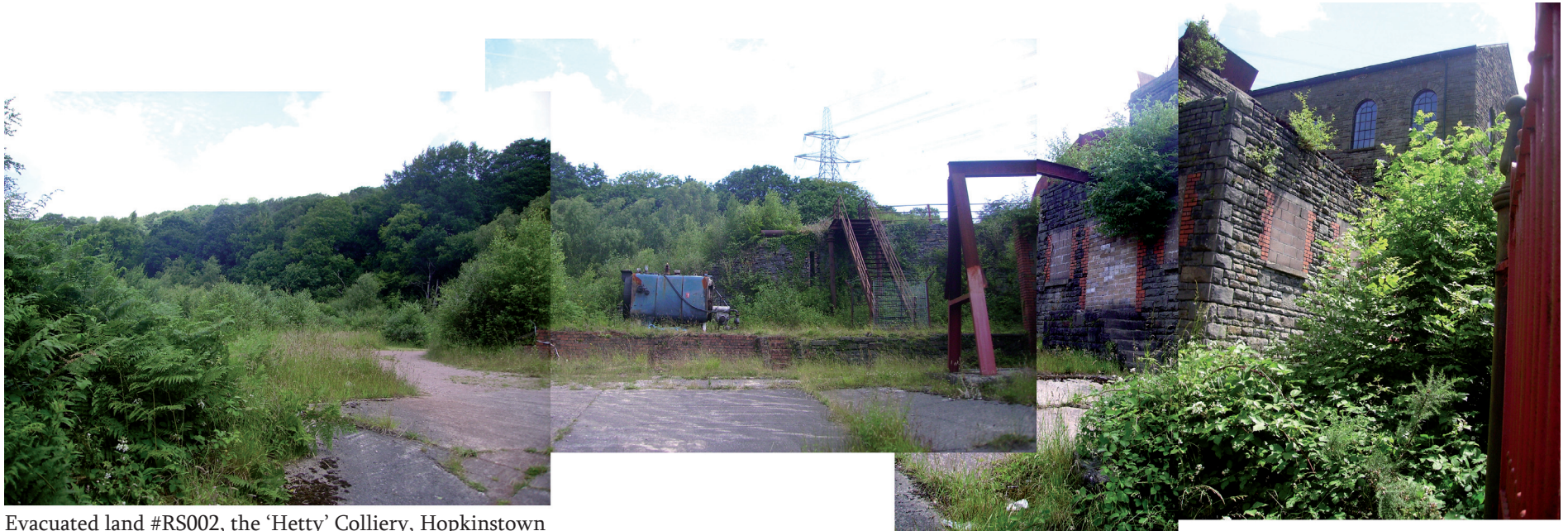
Evacuated land #RS002, the 'Hetty' Colliery, Hopkinstown
