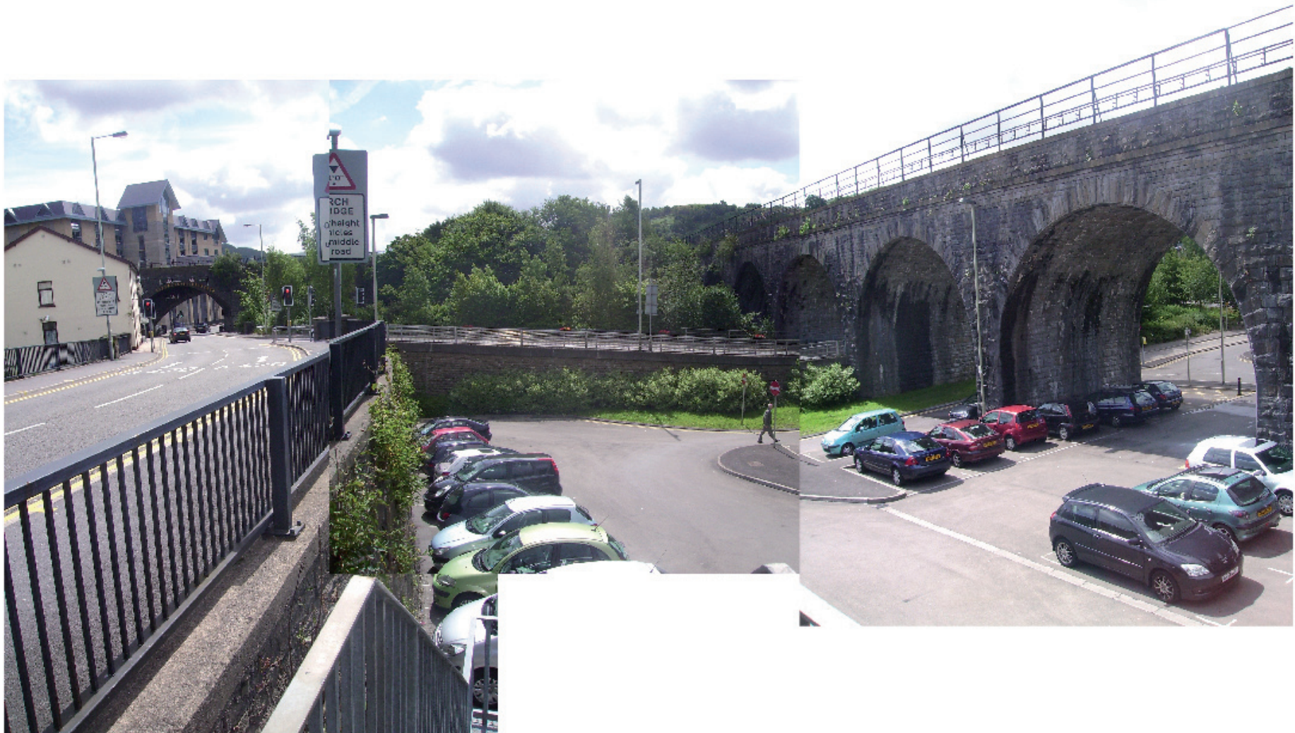
View of #RS001 residual space from adjacent car park
