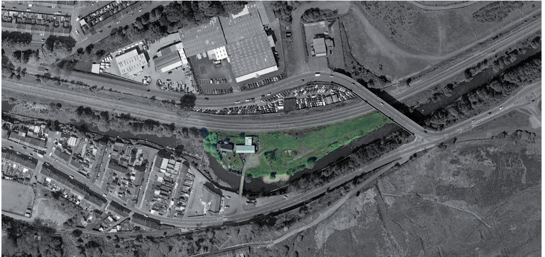
Fig. 4: Aerial view of #RS003 site
