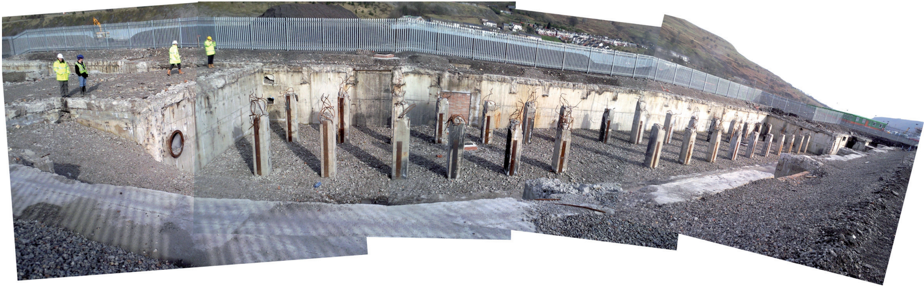
'5 Stand Clean Line', derelict concrete basement structure, 2009
