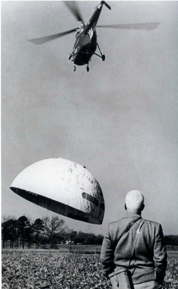
Fig. 10: Helicopter Lifting a Geodesic Dome in Raleigh, 1954. R. Buckminster Fuller.
