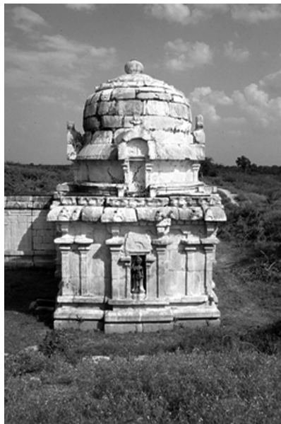
Fig. 18. A Drāviḍa alpa vīmāna (cf. Figure 17c): Bhūmīśvara Śiva temple, Viralur, Tamil Nadu, mid-ninth century. (Photo courtesy of Gerard Foekema)
