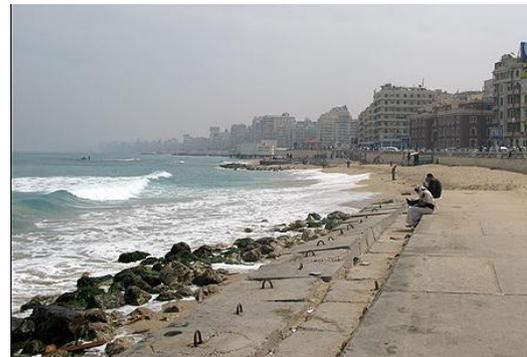
Fig 5 Rising water levels in the Mediterranean Sea are causing the barriers that line Alexandria, Egypt's Eastern Harbour, to slowly break down. (Hansen, 2008 )
