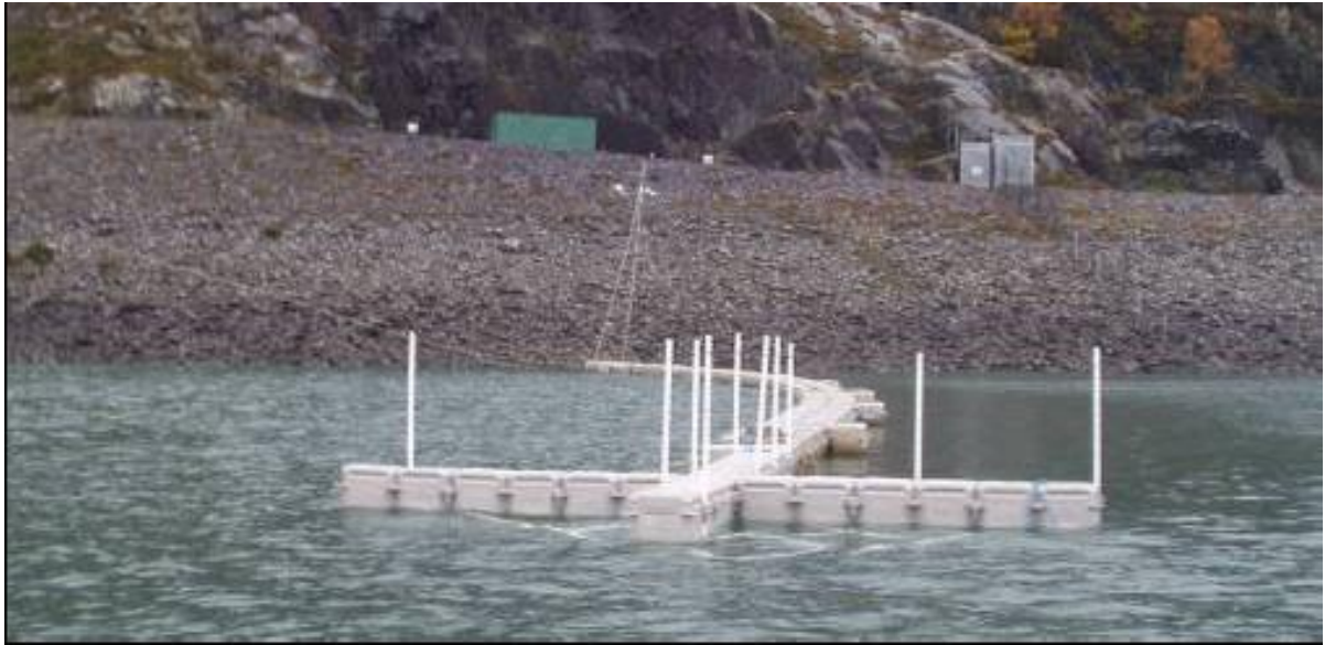
Figure 4.11 View of 5m x 5m grid installed at the far end of the pontoon chain
