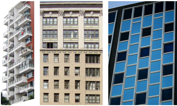
Figure 2: Facades with concatenated grids and/or interlaced grids of architectural elements are ubiquitous in urban scenes.
