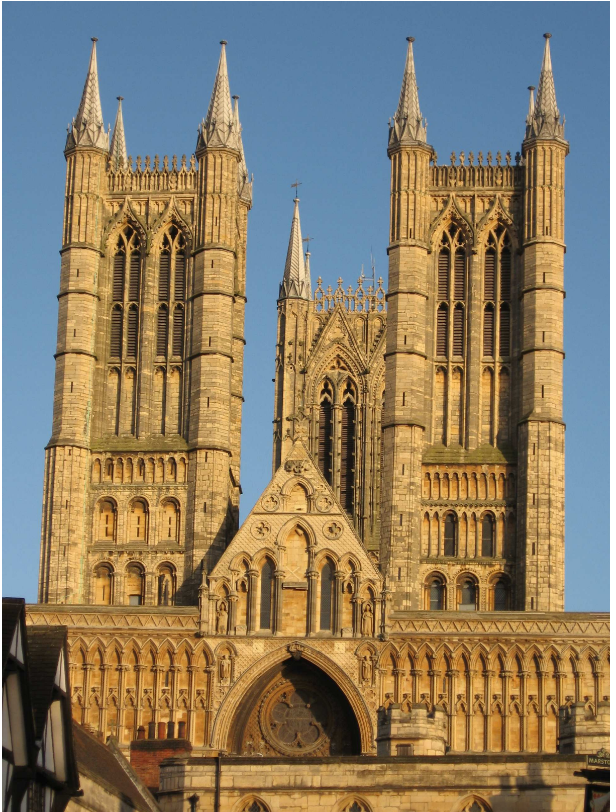
Figure IX: Lincoln Cathedral, façade.
