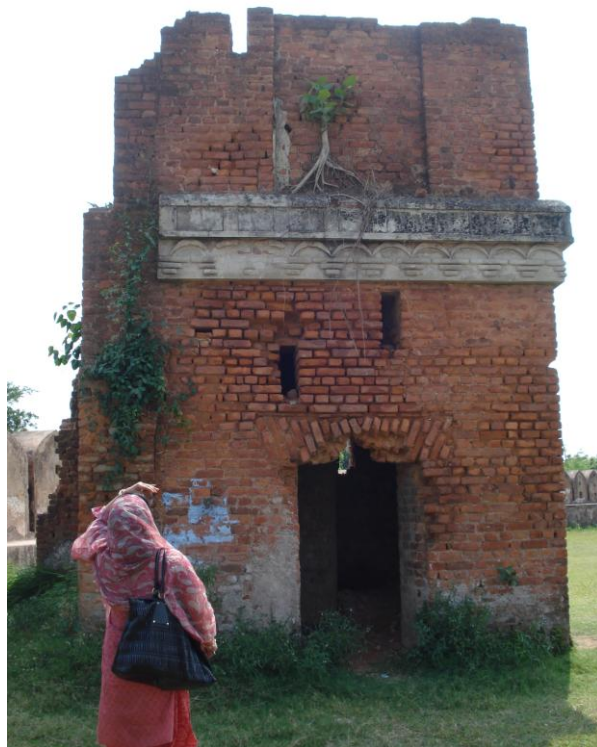
Plate 4 b. Observatory tower of the Hajiganj fort
