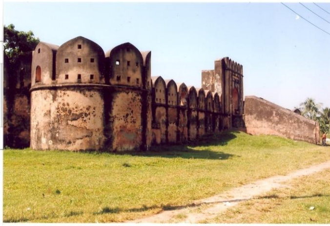
Plate 2 a. Eastern bastion of the Hajiganj fort before renovation (source: the Archaeology Department of Bangladesh)
