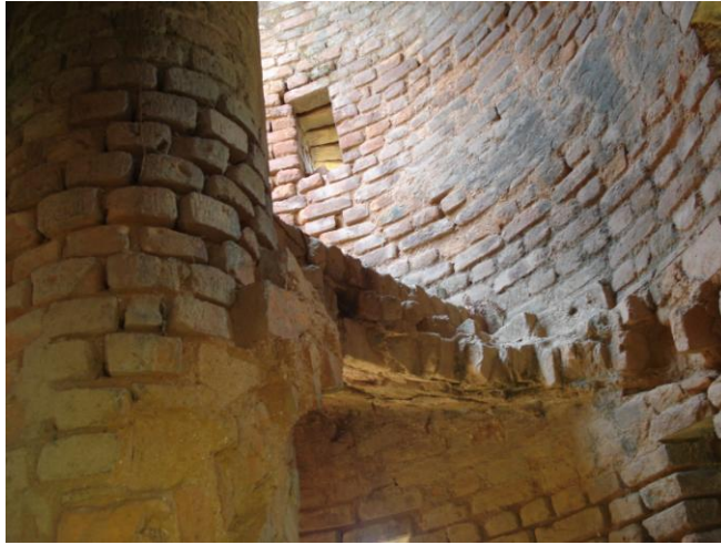
Plate 5 a. Inner pillar with spiral stairs of the observatory tower of the Hajiganj fort
