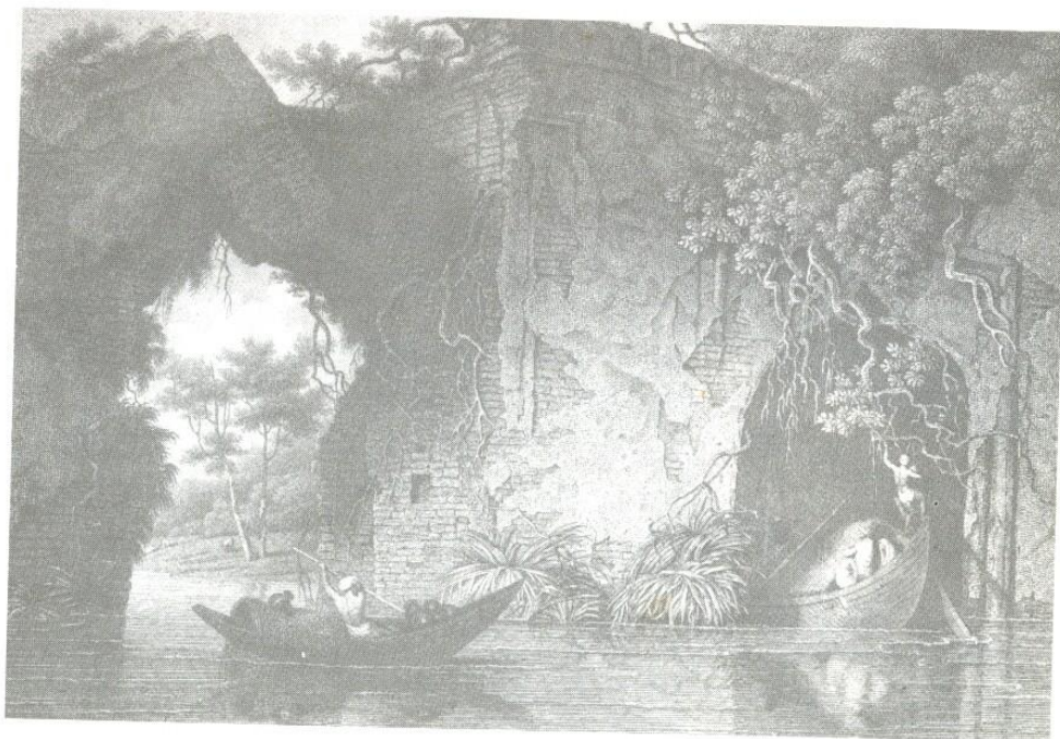
Plate 18 a. Tongi Bridge (Dojly, 1815))
