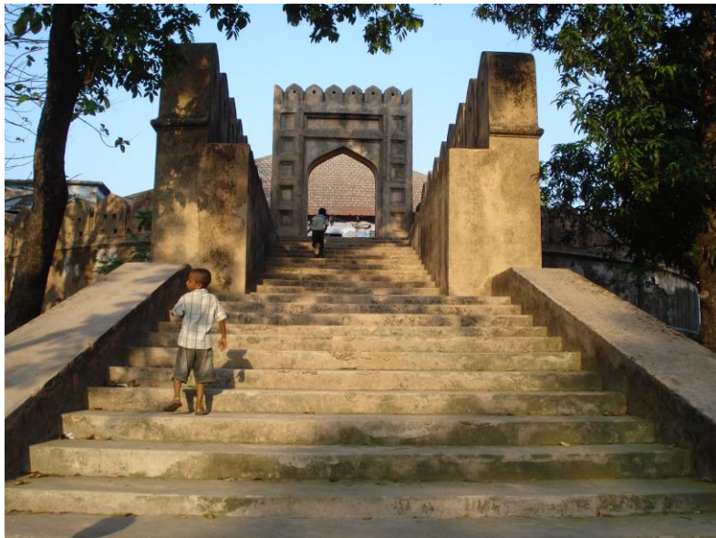
Plate 11 b. Stairs of the observatory tower of the Idrakpur fort
