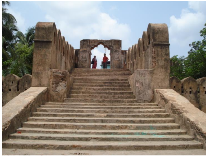
Plate 7 a. Stairs of the observatory tower of the Sonakanda fort
