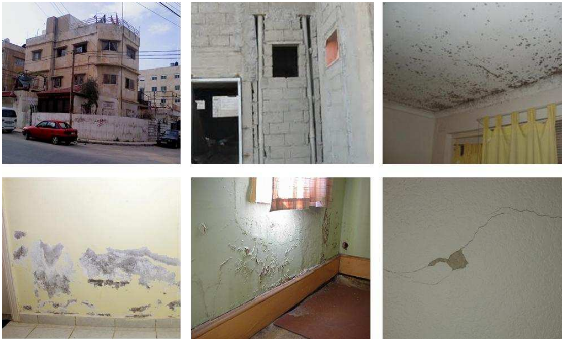
Figure 8.13: Examples of some common deficiencies in the quality of construction
