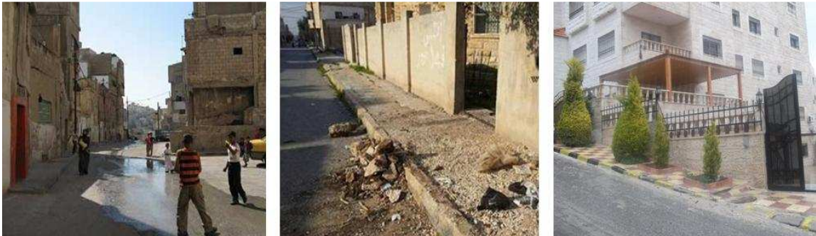
Figure 7.12: Examples of deficiencies in infrastructure in some locations
