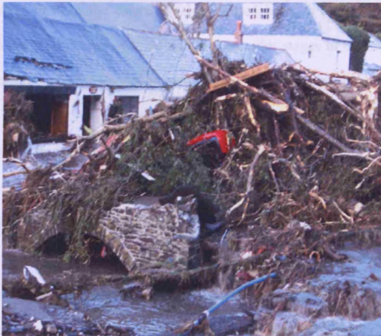
Figure 6.4 The Lower Bridge blocked by vehicles and other large debris during 2004 Boscastle flood (Photograph courtesy of www.tintagelweb.co.uk )
