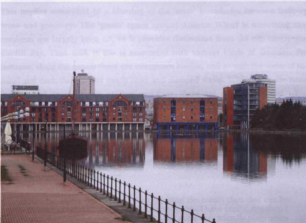
Figure 6.3 The Bute East Dock
