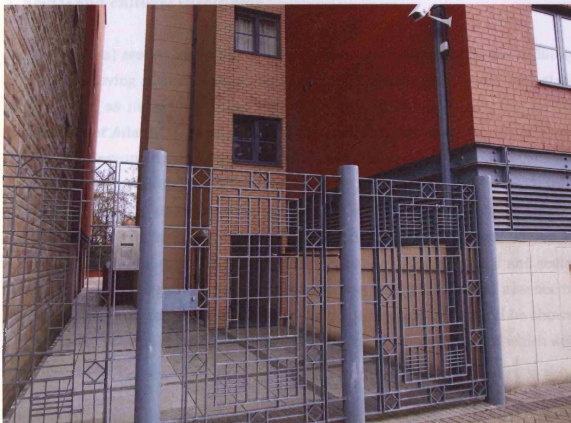
Figure 6.4 The Granary, a secure gated development on Lloyd George Avenue
