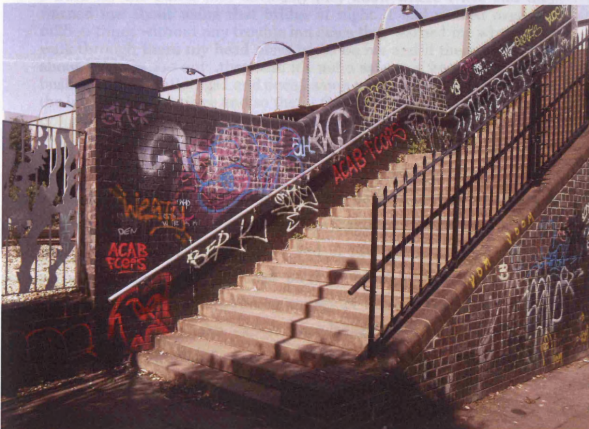
Figure 7.5 Pellett Street footbridge
