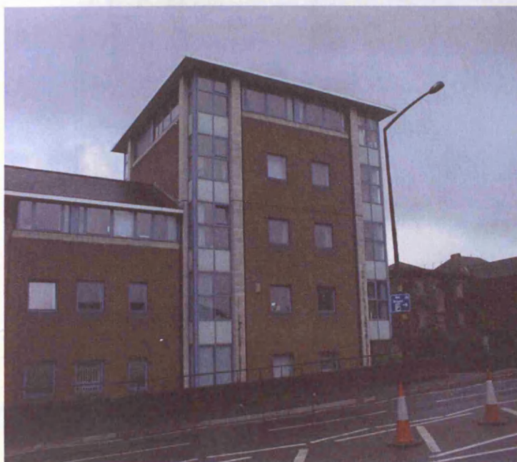
North Facade of Building
