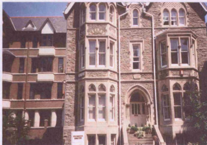
Link to Existing Building (retained, older facade)
