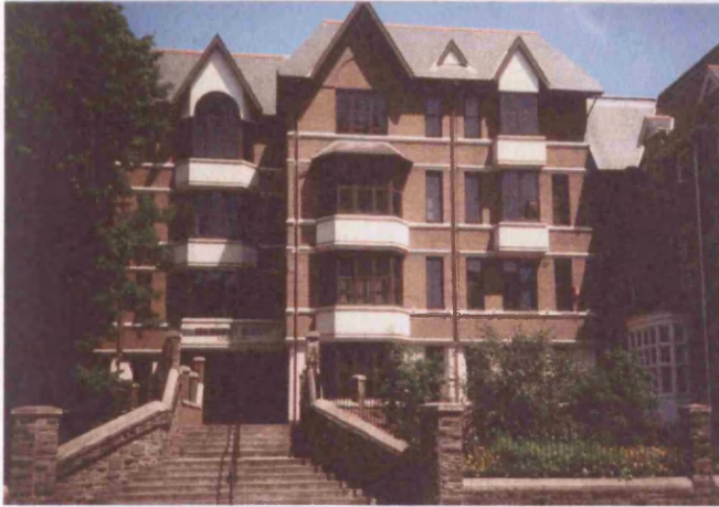
New Building - West Facade of Building
