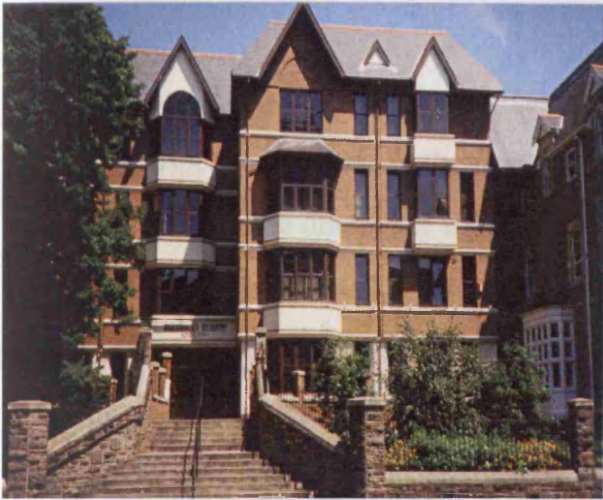
Front View of Building
