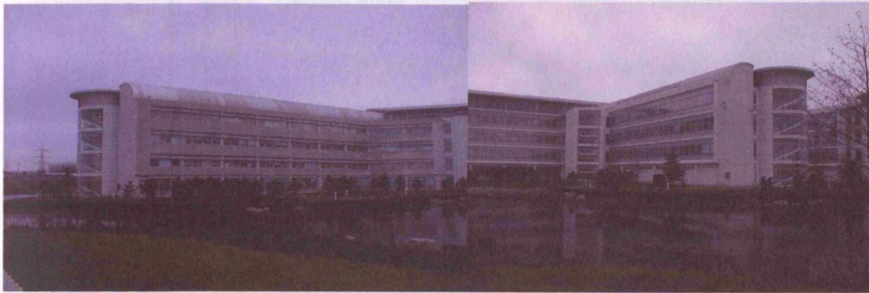
South Facing Facade of Building
