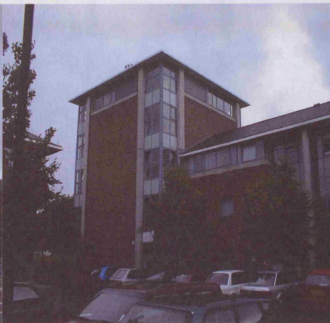
South Facade of Building
