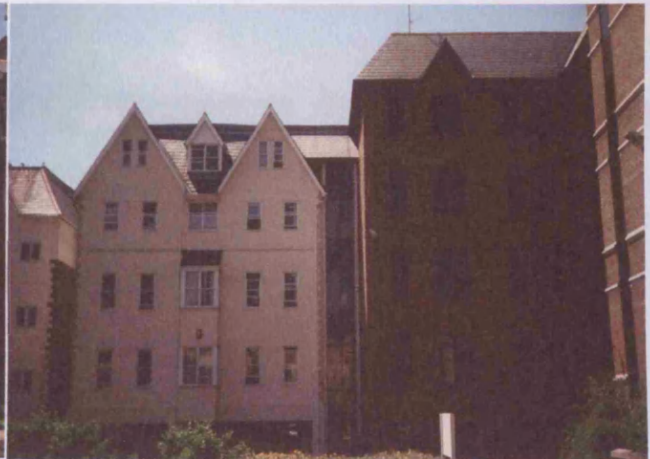
New Building - East Facade of Building
