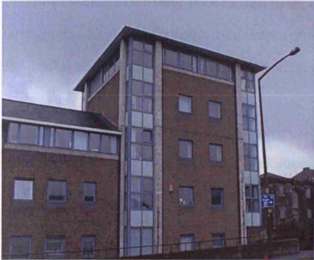
Front View of Building
