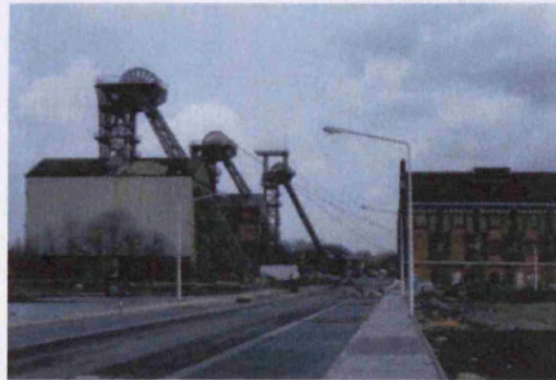
Fig. 6.7 - D Fig. 6.6 - Listed shaft towers (view to the north-east)
