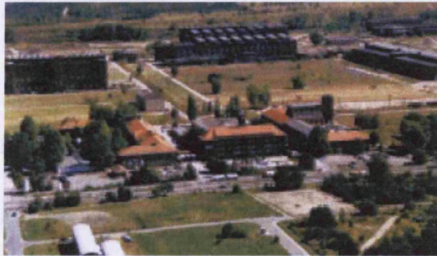
Fig. 6.9 - Eastward aerial view of the site
