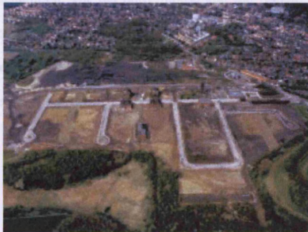
Fig. 6.5 - Northward aerial view of the site
