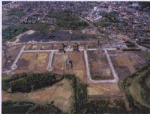
Fig. 6.5 - Northward aerial view of the site
