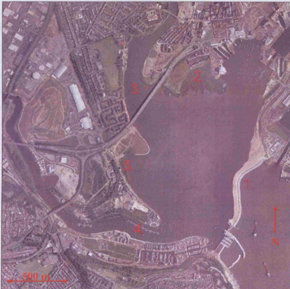
Figure 2.4: Aerial photograph of Cardiff Bay (post-barrage) showing numbered points of interest: 1) Cardiff Bay Barrage; 2) Cardiff Bay Wetland Reserve (Windsor Esplanade); 3) River Taff estuary; 4) River Ely estuary; 5) Former Salt Marsh (Prospect Place).
