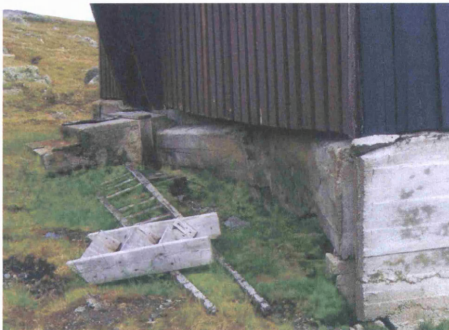
Figure 1.3.1. The impact of gelifluction on the concrete foundations of a small mountain building, Finse, Southern Norway (Photograph: Ivar Berthling).
