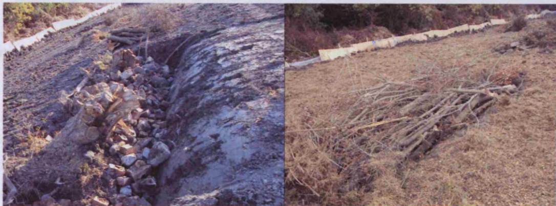
Figure A4.3 The hibernacula foundation is filled with rocks (left) to a height of 1-2 m and then insulated with a 1 m layer of recycled branches and roots (right).
