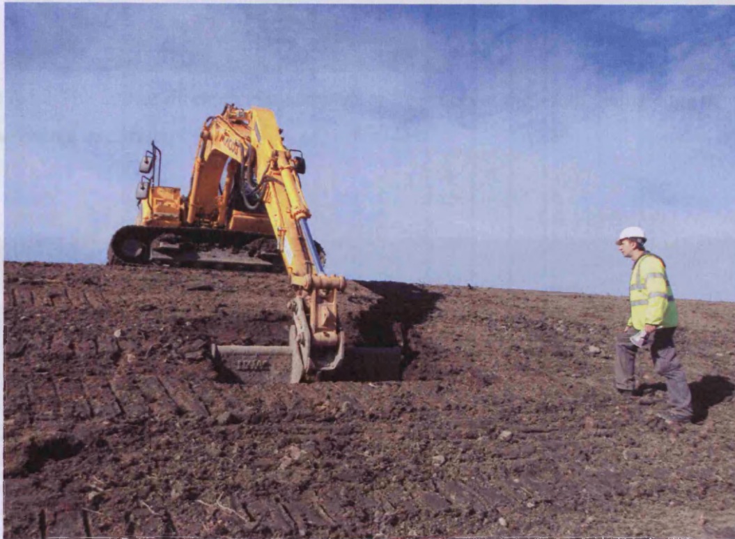
Figure A4.1 The author supervising a 16 tonne digger as it excavates the base of the hibernacula at the receptor site.
