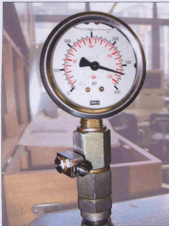
Figure 3.5: Pressure testing the pressure transducer fitment
