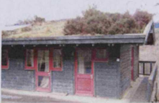
Figure 38. Simple intensive green roof in the Centre for Alternative Technologies, in Machynlleth (author)
