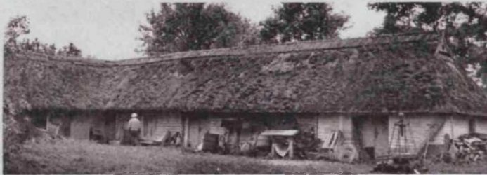
Figure 96. Outbuildings under one, turf roof, in the Island of Muhu, in the Baltic area (Oliver, 1997c)
