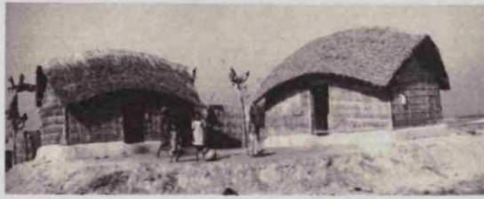
Figure 74. Namoshudra dwellings with curved thatched roofs in Bangladesh (Oliver, 1997c)
