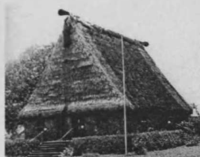
Figure 54. A Fijian chief's house with thatched roofs, on elevated platform (Oliver, 1997c)
