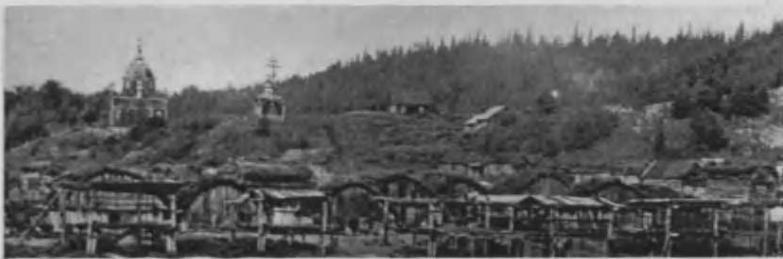
Figure 101. Multi family vertical log dwellings with sod roofs on the banks of the Yukon River, Alaska (Oliver, 1997b)
