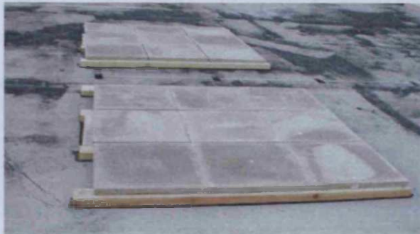
Figure 155. Slabs on the top of timber frames for both “concrete” and “green” test cells
