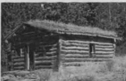
Figure 102. Miner's turf roofed log house in Wallahachin, Thompson river valley (Oliver, 1997b)
