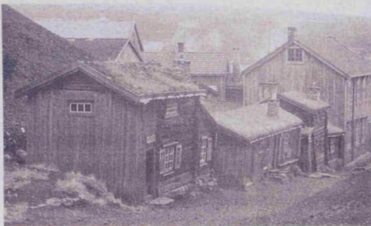
Figure 98. Miners' houses with turf roofs dating from the 17 th to the 19 th century in Røros, in Sør-Trøndelag, Scandinavia (Donnelly, 1992)
