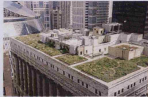
Figure 135. The green roof of the City Hall of Chicago (Laberge, 2001)
