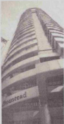
Figure 41. Yeang's Boustead building in Malaysia, with plants hanging from the balconies as "curtains" 10 (Yeang, 1992)
