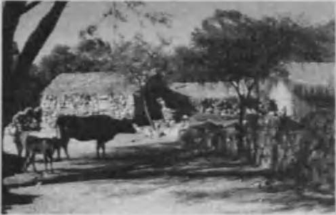
Figure 72. Thatched roofs on stone walls in typical Quechua dwellings (area between Argentina, Bolivia and Chile) (Oliver, 1997c)
