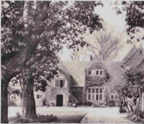
Figure 123. Letchworth Hall with its ivy-covered wall, in the early 1930s (Miller, 2002)
