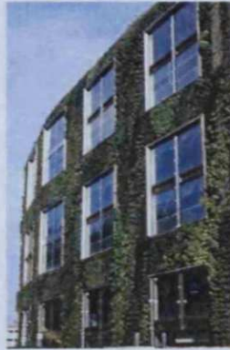
Figure 119. View of Patrick Blanc's newly formed (summer 2004) "mur végétal" in the Musée du Quai Branly (Musée du Quai Branly, 2004)
