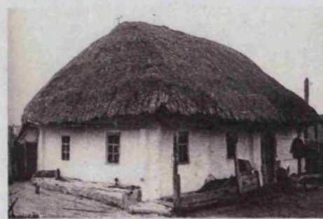
Figure 91. Early 20 th century house with thatched roof in Kursk Province, south Russia (Oliver, 1997c)
