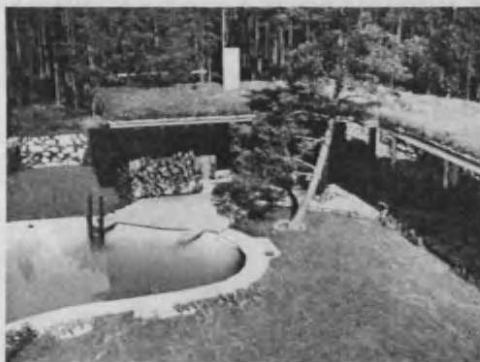
Figure 111. Sod roofs by Alvar Aalto, on the sauna of the Villa Mairea (Curtis, 1982)
