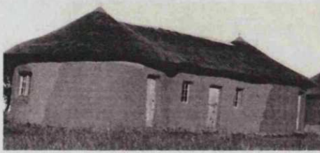
Figure 62. Linked cone-on-cylinder Xhosa house with thatched roofs in Cape Nguni in Southern Africa (Oliver, 1997b)
