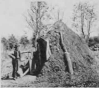
Figure 94. Charcoal burner's hut covered with earth and grasses in England (source: www.yeoldsussexpages.co.uk )
