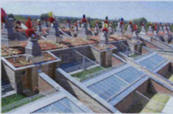
Figure 132. View of green roofs in BedZED [source: http://www.zedfactory.com ]
