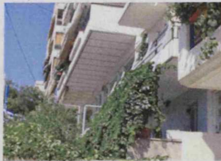
Figure 42. Green wall adjusted to the building with a metal frame, creating an intermediate exterior living space, protected from the summer sun, in Athens (author)
