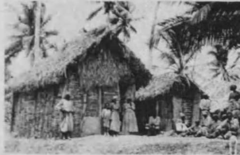
Figure 73. Nineteenth-century huts with thatched roofs and reed or wood walls in Saint Elizabeth, Jamaica (Buisseret, 1980)
