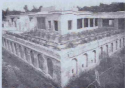
Figure 48. The reconstructed green roofs at the ruins of the Villa of the Mysteries in Pompeii (Jashemski, 1979)
