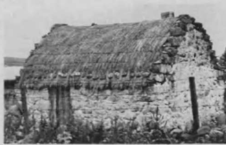
Figure 95. Simple thatched roof in Ireland (Kahn, 1973)
