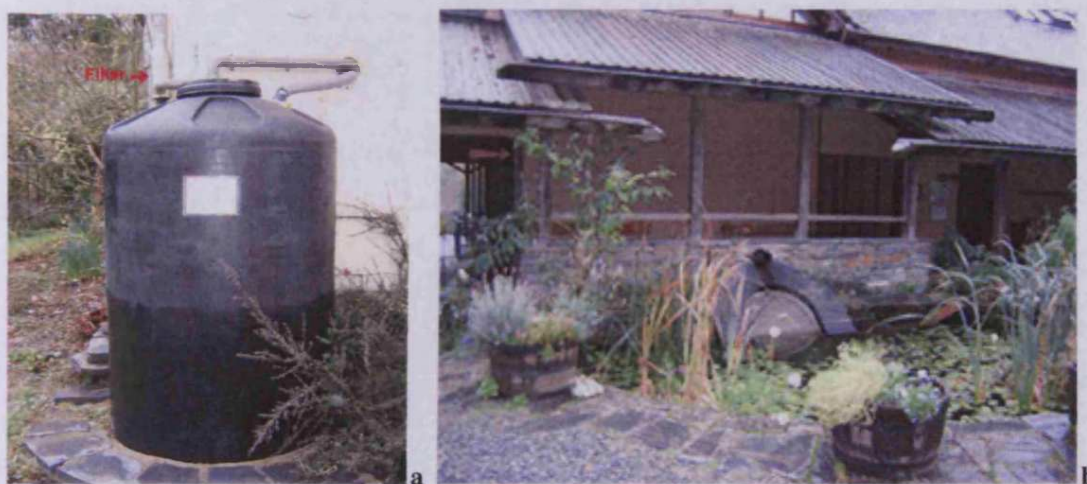
Figure 3. Rainwater reservoirs in the Centre for Alternative Technologies; (a) closed tank with filter and (b) pond (open reservoir) with aquatic ornamental plants (author)
