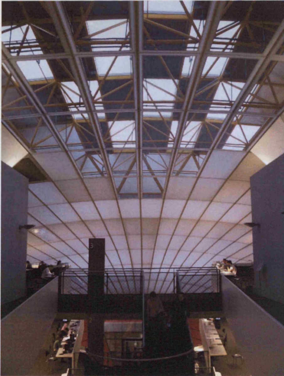
Fig.128 Interior of the Philological library. The curving skin of the 'bubble' can be seen revealing yellow painted steel structure in the interstitial space between interior and exterior skins
