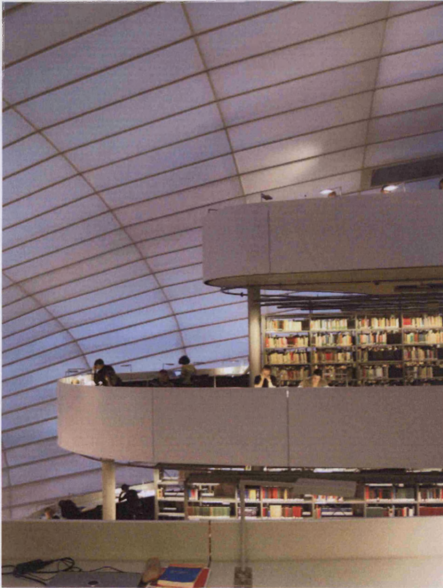
Fig.130 Interior of the Philological library. The curving skin of the 'bubble' can be seen revealing yellow painted steel structure in the interstitial space between interior and exterior skins
