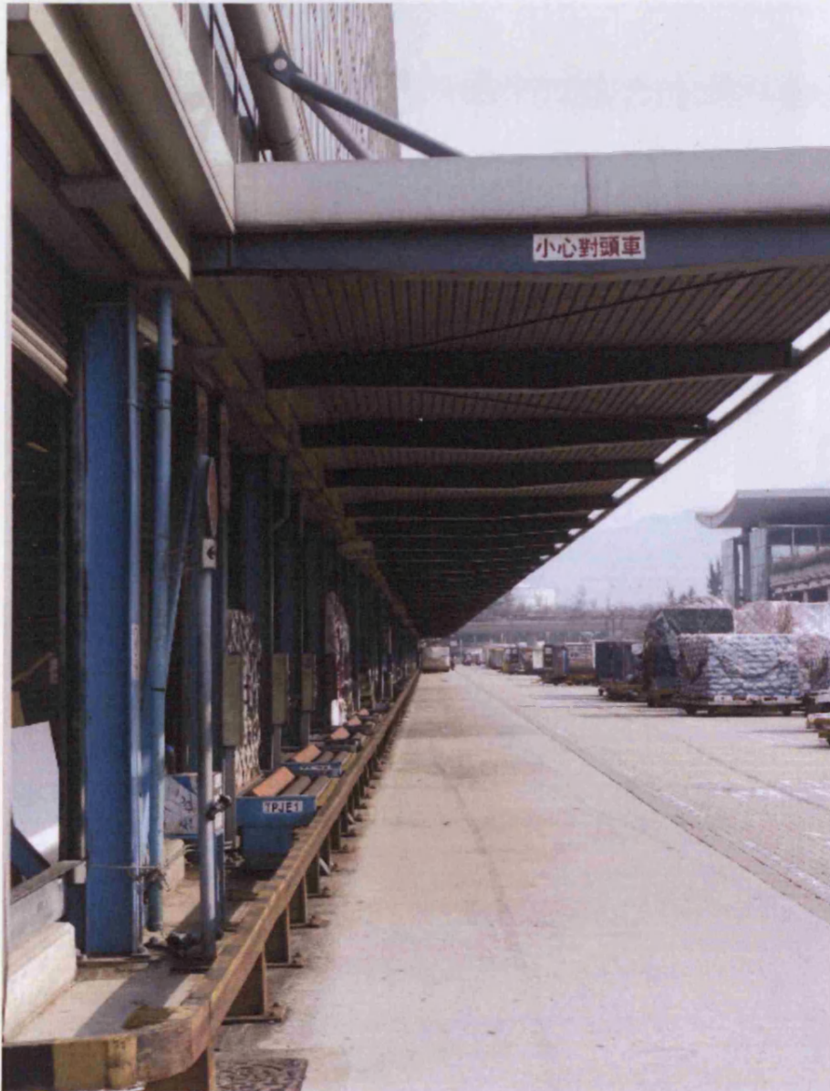
Fig.107 Cargo interface: the Express Cargo Centre is visible in the back-right of the photograph
